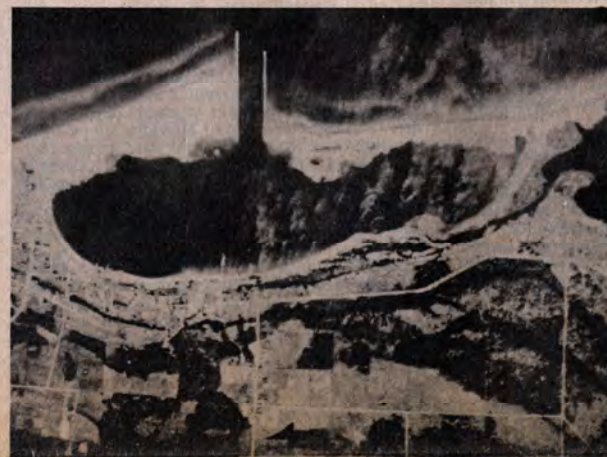
The above U.S. Army Corps of Engineers' map details the Grand Marais Harbor. The pile dike stretching across has been in disrepair. Efforts are now moving at achieving state and federal funding to rebuild the dike. Left, a 1939 aerial photo of the Grand Marais Harbor and pile dike.
