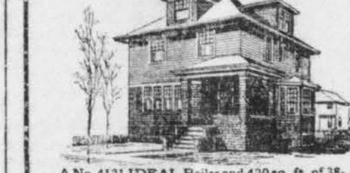
A No. 4121 IDEAL Boiler and 420 sq. ft. of 38" AMERICAN Radiators, costing the owner $195, were used to heat this cottage. At this price the goods can be bought of any reputable competent fitter. This did not include cost of labor, pipe, valves, freight, etc., which vary according to climatic and other conditions.
