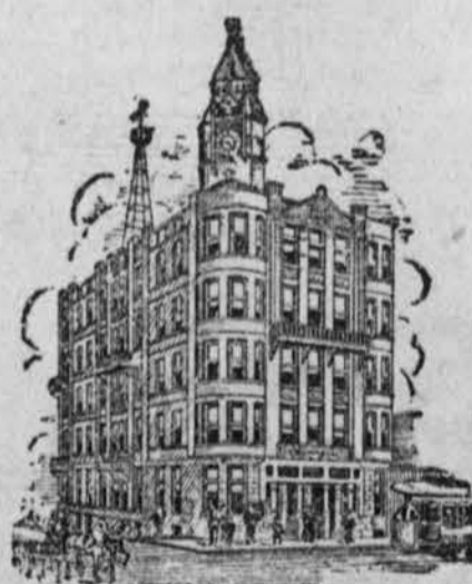
Savings Bank Building, owned by Marquette County Savings Bank.
