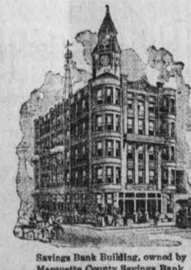
Savings Bank Building, owned by Marquette County Savings Bank
