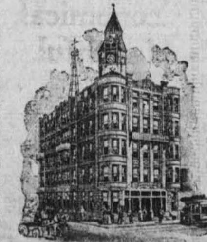
Savings Bank Building, owned by Marquette County Savings Bank
