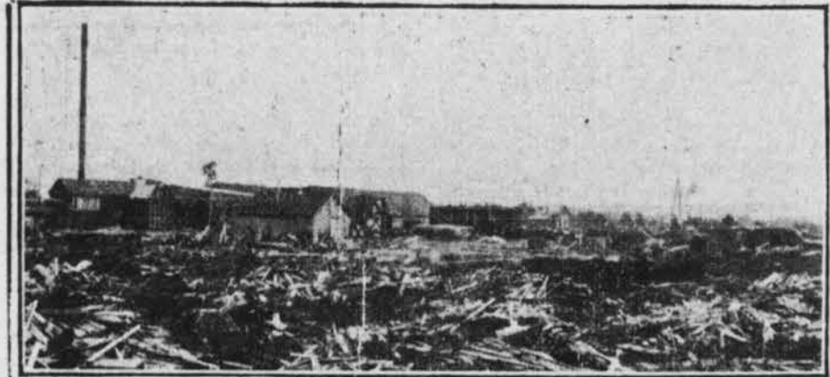
General View of B. J. Goodman & Son's Little Lake Saw Mill.
