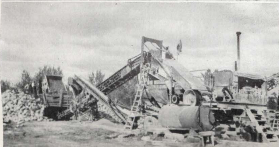
Menominee County's Gravel-Crushing Plant — Daily Capacity, 600 Cubic Yards
