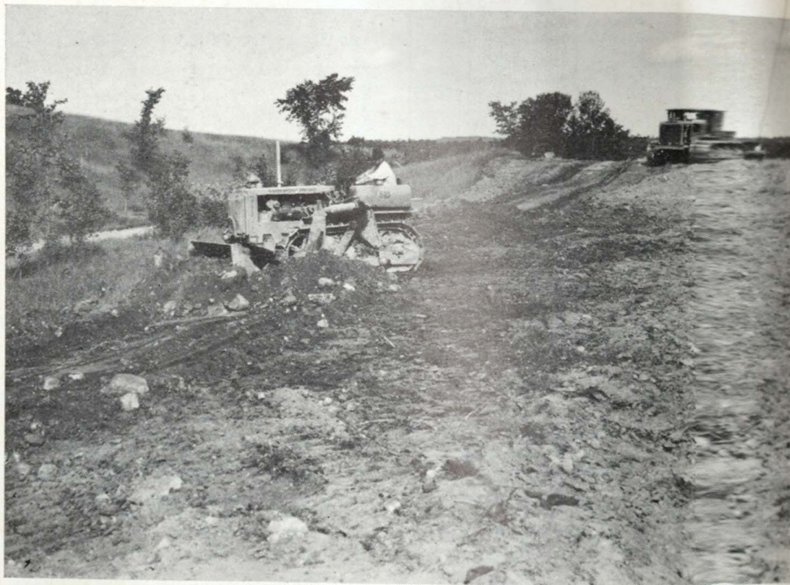
Bull-Dozer Levelling a Hump in the Road
