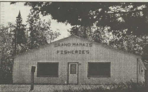
C-120 The Grand Marais Fisheries building is over 2400 square feet with many possibilities, waiting for your idea to open a business. Located east of town on H-58 with a separate one bedroom cabin. $140,000
