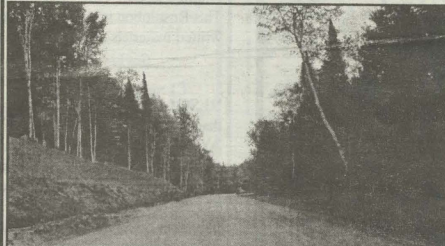
Above, once an extremely steep hill, this section now cuts through the peak and provides a long, gentle slope.
