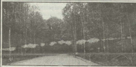
Merging back into the original roadway.
