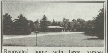
Renovated home with large garage/workshop area on 10 acres, year around access. Ideal for snowmobilers.
