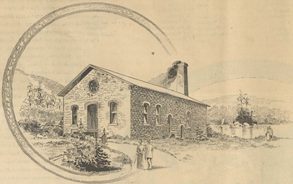
CITY WATER WORKS ENGINE HOUSE.
