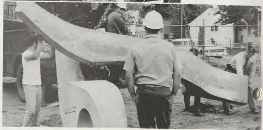
Professor Wolfram Niessen, Art, and his sculpture students spent long summer hours constructing the concrete statuary that appears in several spots on Northern's campus.
