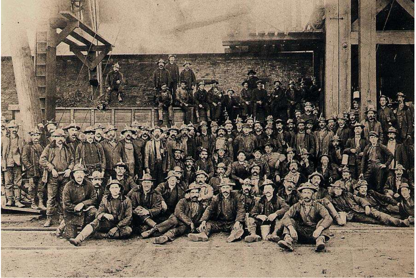
This unidentified group of miners wearing miner's candlesticks on their mining hats probably dates between 1890 and 1900. Note the huge timbers of the mine shaft at the right.
