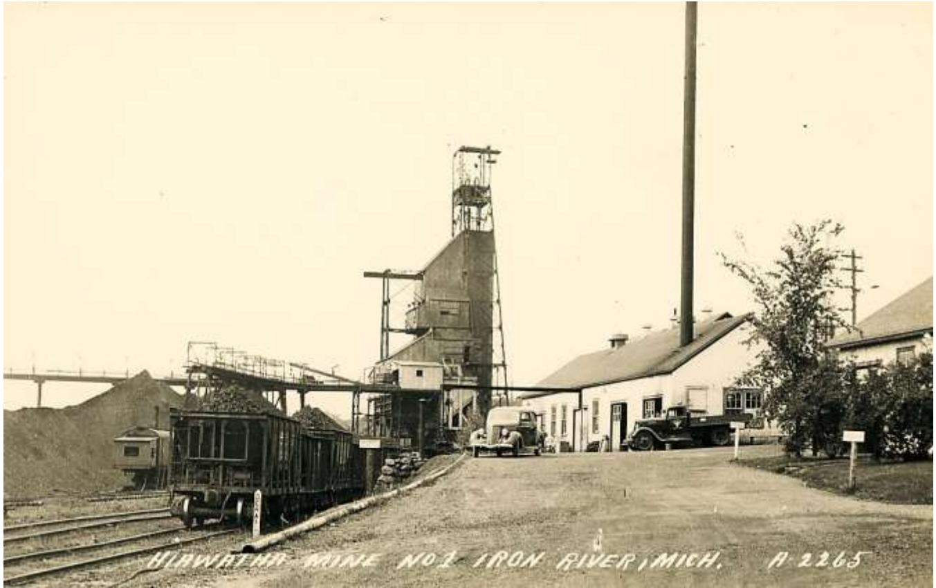
Hiawatha Mine No. 1, Iron River, Mich. A-2265 , (showing Hiawatha Mine No. 1 with shaft housing, mining buildings, loaded ore cars and stockpiles at extreme left) unused (real photo, EKC 1940-1950) [2013 – Dave Jaeger, Haslett, MI – $11.95] $15.00
