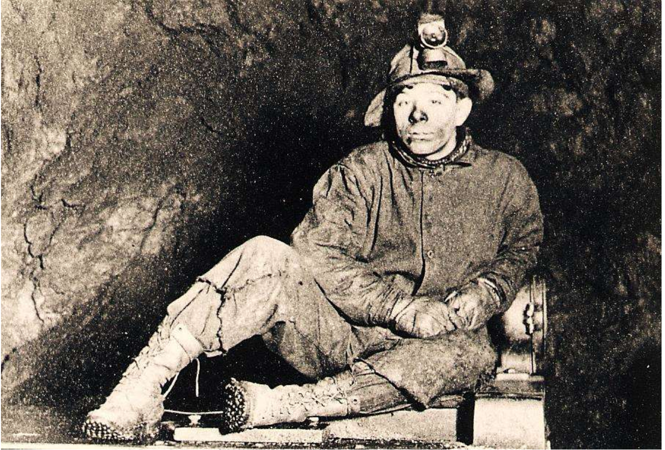
This unidentified miner posed on a piece of mining equipment underground. Note the carbide lamp on his mining hat and the clogged boots. [William J. Cummings]
