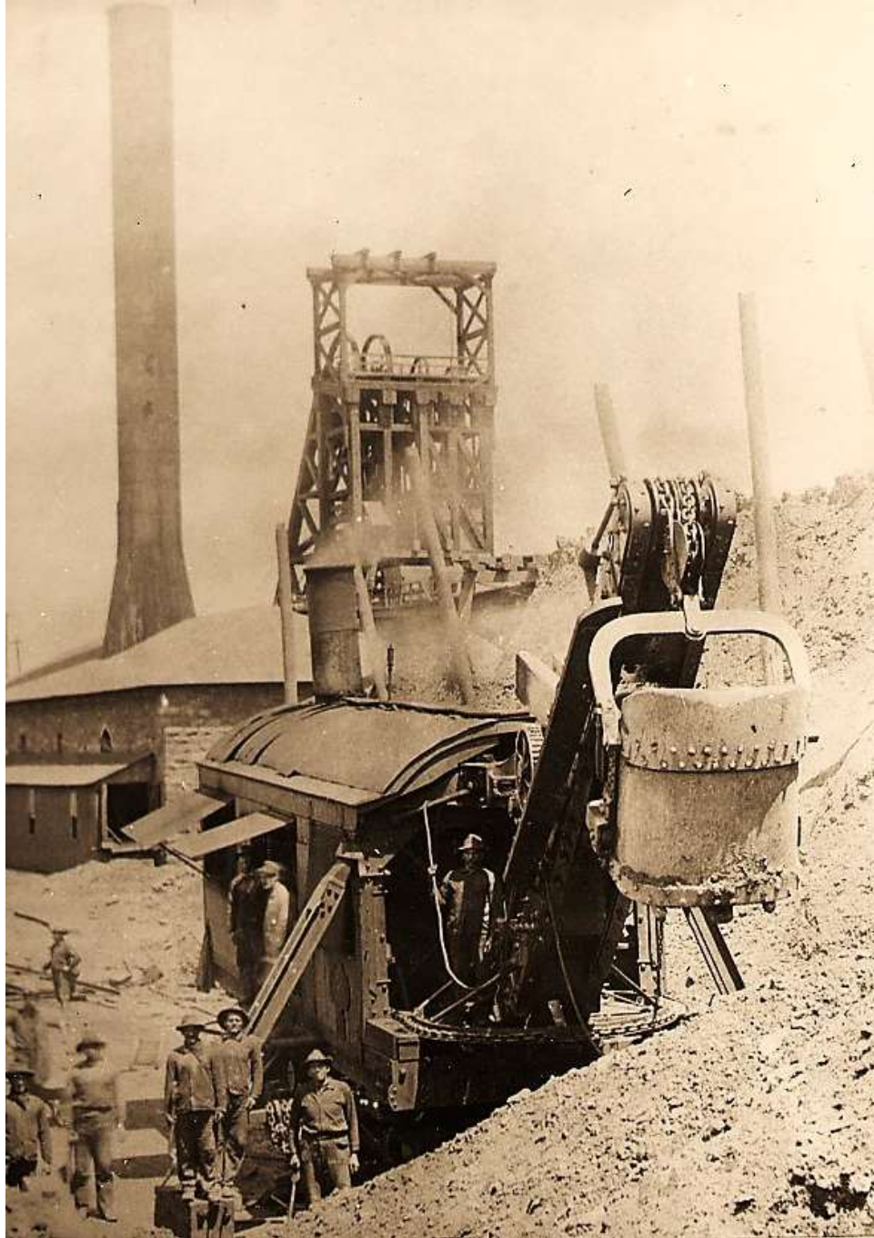
The steam shovel was an expensive and vital piece of machinery, particularly for the larger mining companies, and was used to load stockpiled iron ore into the railroad cars. The steam shovel and crew of the Hamilton Shaft of the Chapin Mine are pictured here in about 1900. [Menominee Range Historical Museum]
