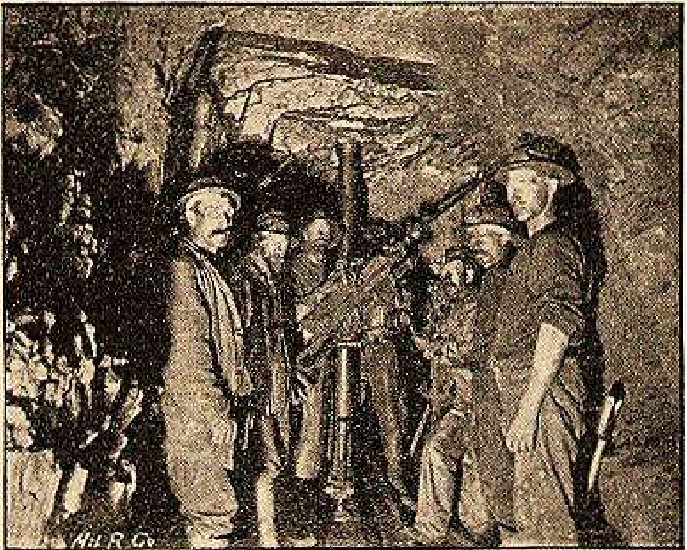
RAND DRILLS—4TH LEVEL LUDINGTON MINE.
