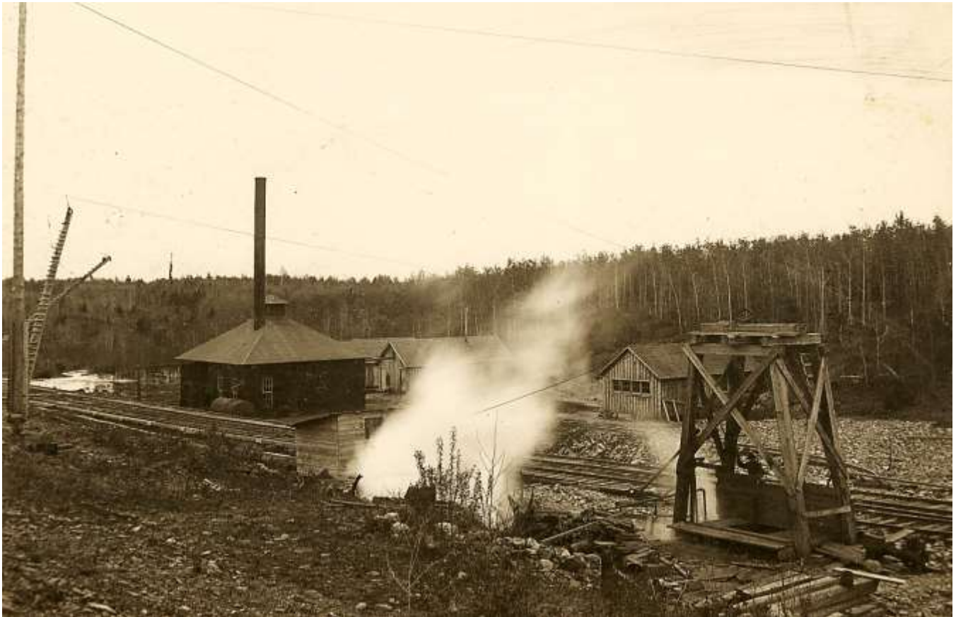
This view of the Keel Ridge Mine was taken by Jorgen J. Eskil in 1900.
