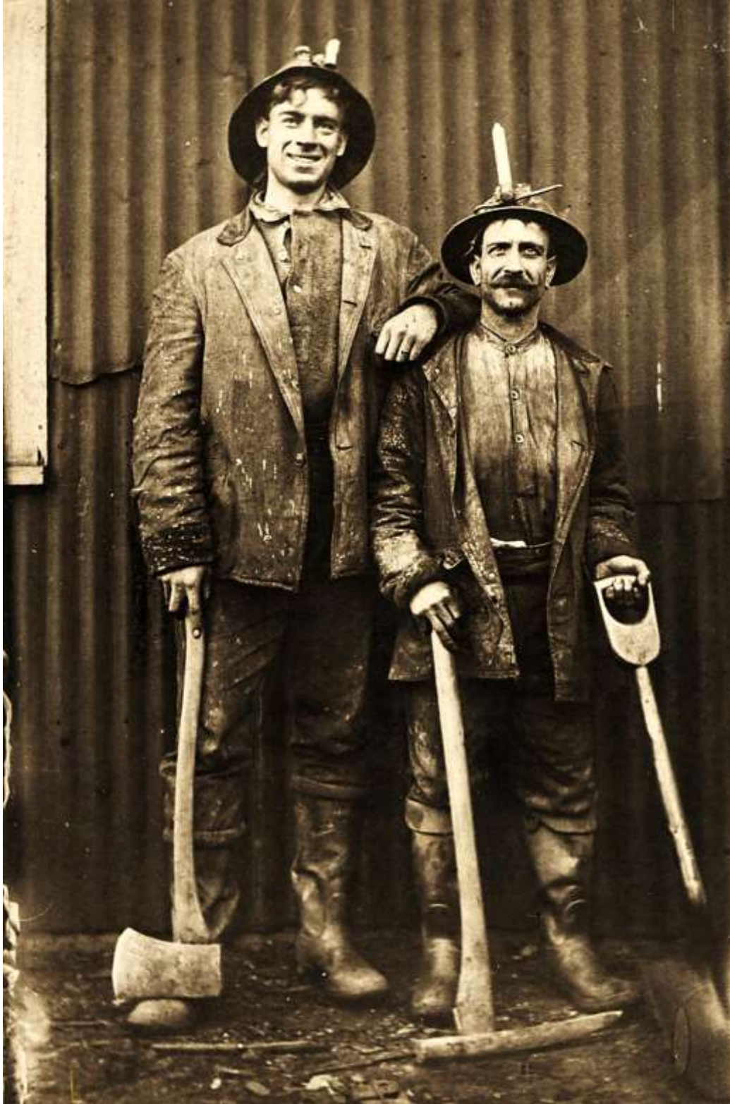
William Joseph Trestrail (left) and his Italian mining partner, wore oilskin clothing and rubber boots to protect them from the wet conditions at the Pewabic Mine in about 1910. Note the miner's candlesticks in their hats which provided illumination for work in the mine. [Menominee Range Historical Museum]
