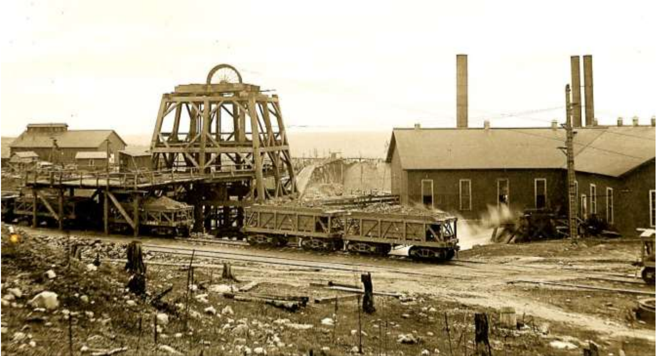
This view of the Pewabic Mine, showing the wooden shaft housing, was taken by Jorgen J. Eskil, pioneer Menominee Range photographer, in May, 1899. [Menominee Range Historical Museum]
