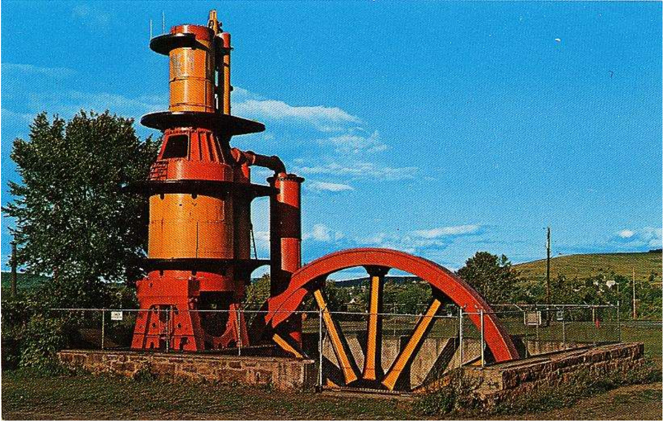
Painted orange and yellow-gold with black trim, this unused postcard view of the “Cornish Mine Cornish Pumping Plant” probably dates between 1960 and 1970. [William J. Cummings]
