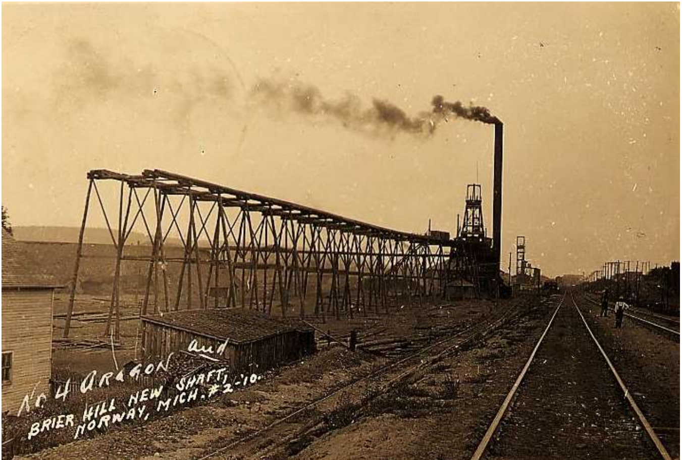
Postmarked Norway, Mich., October 8, 1910, this postcard view, taken in 1910, shows No. 4 Aragon and the new Brier Hill Shaft, looking east. Railroad Street would be at the right on the other side of the railroad tracks. [William J. Cummings]
