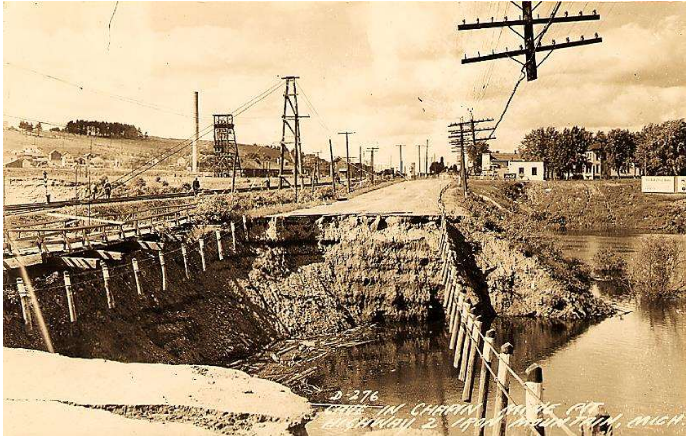
Another postcard view shows a close-up of the cave-in with debris floating in the water. [William J. Cummings]
