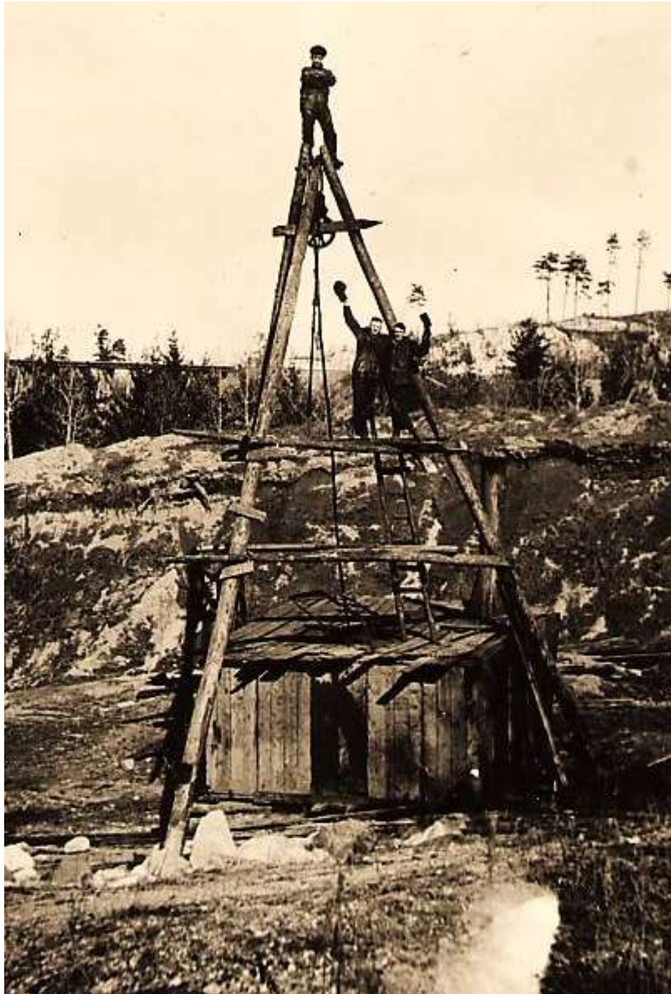
This photograph shows a diamond drilling rig set up on the McKenna property near Fumee Creek. The railroad bridge is visible in the background at the left. Walter Alquist, Axel Alquist and Amie LaPoint are the men on the diamond drill rig. [John Alquist]
