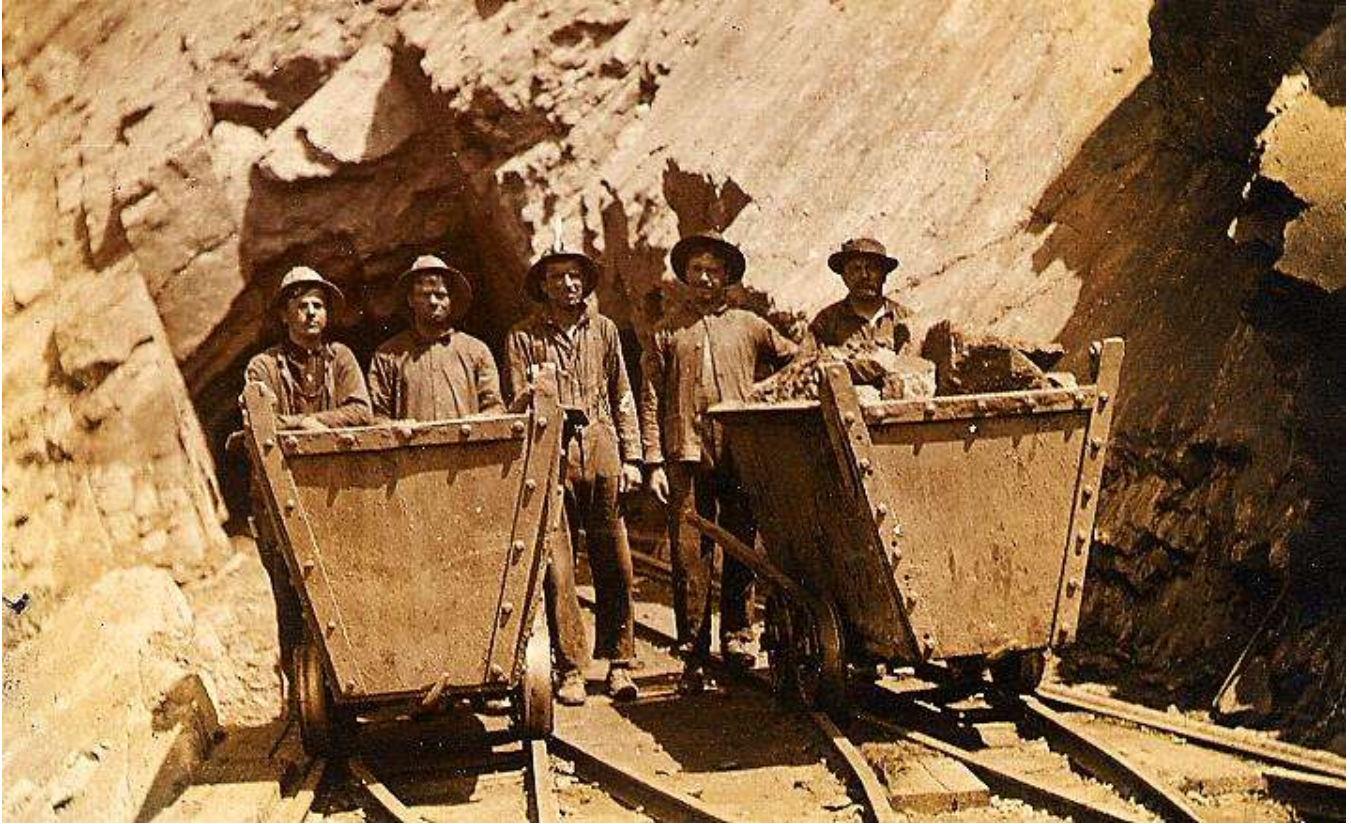
Postmarked Iron Mountain, Mich., July 27, 1908, these five trammers posed with two tram cars loaded with iron ore in what may be the entrance to the Quinnesec Mine. [William J. Cummings]
