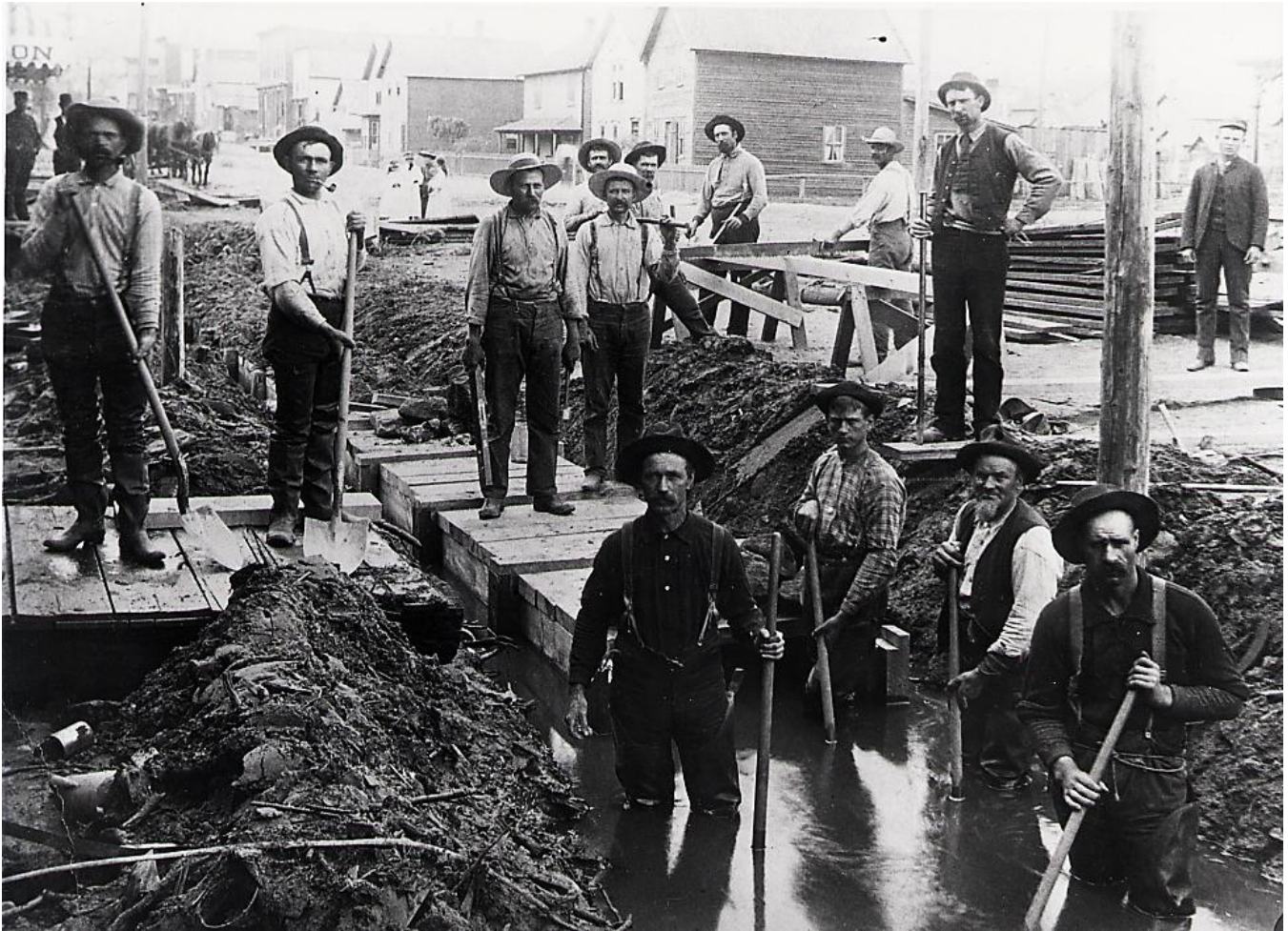
Northwest Corner of Carpenter Avenue and West Hughitt Street, Iron Mountain, June, 1891: Workmen were boxing in the mine creek which ran along the side of Iron Mountain's West Hughitt Street from Merritt Avenue west in mid-June, 1891, to "prevent children from throwing debris into the water," according to The Iron Range . The camera faces east, and this unidentified city crew was working at the northwest corner of Carpenter Avenue and Hughitt Street. Buildings on the south side of the street are visible behind the workers. [ Menominee Range Historical Museum ]
