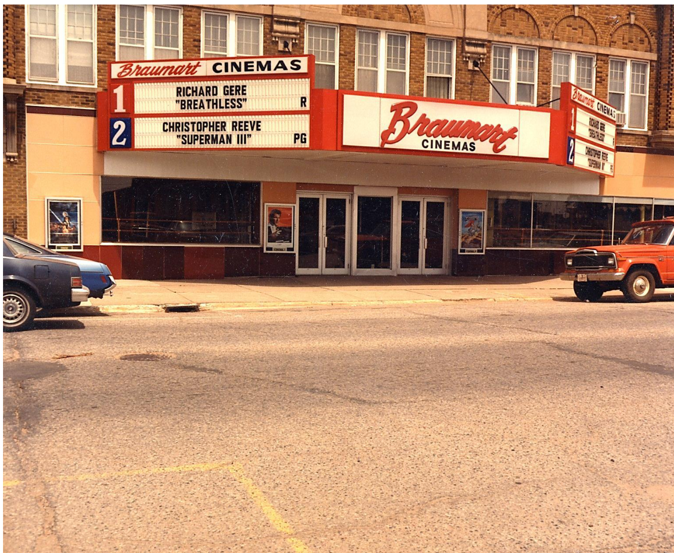
The Braumart Cinemas, 104-108 East B Street, Iron Mountain, 1983: The Braumart Theater's auditorium was divided into two parts in 1982. In 1983 "Breathless," starring Richard Gere, and "Superman III," starring Christopher Reeve, were listed on the marquee. Note that the ticket booth was no longer between the two sets of double doors, and the red "Braumart" had replaced the lighted version. [Tom and Liz Renn]
