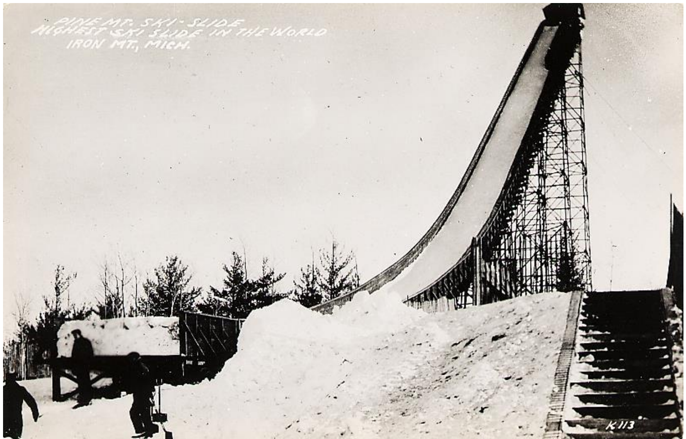
K-113 Pine Mt. Ski Slide, Highest Ski Slide in the World, Iron Mt., Mich., ca. 1940-1950: This unused postcard view, taken from the cement stairway going up the hill to the scaffold of the Pine Mountain Ski Jump between 1940 and 1950, shows workers at the end of the scaffold. [William John Cummings]
