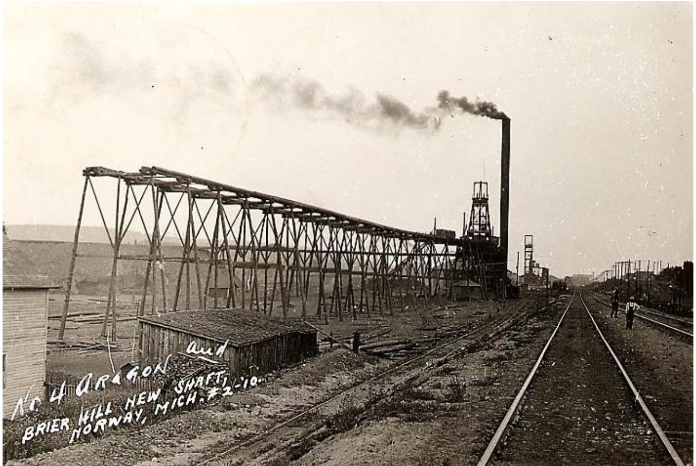
Aragon Mine No. 4 Shaft and Brier Hill New Shaft, Norway, 1910: Postmarked Norway, Mich., October 8, 1910, this postcard view, taken in 1910, shows No. 4 Aragon and the new Brier Hill Shaft, looking east. Railroad Street would be at the right on the other side of the railroad tracks. [William John Cummings]
