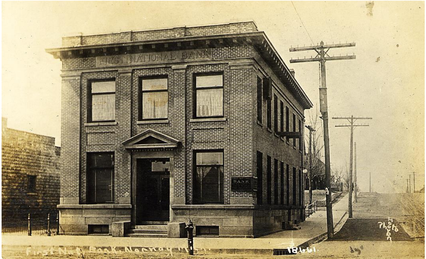
First National Bank, 400 South Nelson Street (Main Street), Looking West, Norway, ca. 1916: Postmarked Vulcan, Mich., September 11, 1916, Norway's First National Bank building was erected at 400 South Nelson Street in 1908. John S. Lindsley, of Escanaba, secured the contract with a bid of $10,450, excluding the vault and plumbing. The two-story brick structure housed the bank on the first floor and office space for rental purposes on the second floor. [William John Cummings]
