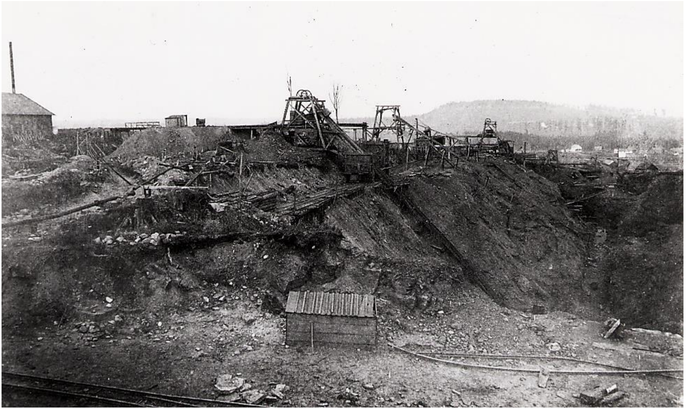
Norway Mine, NE ½ of the SE ¼ of Section 5, T39N, R29W, Norway, May, 1886: Taken in May, 1886, this view, looking east, shows part of the Norway Mine, located on the NE ½ of the SE ¼ of Section 5, T39N, R29W. The Norway Mine was one of the few Dickinson County mines worked as an open pit. [Marquette County Historical Society]
