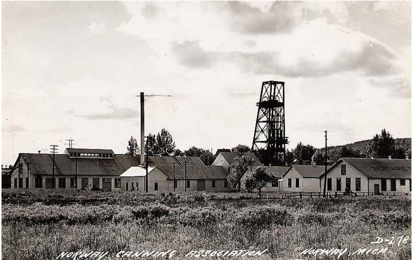
Norway Canning Association, North End of Stephenson Street, Norway, ca. 1930: The Norway Canning Association was located at the north end of Stephenson Street in buildings formerly used by the Aragon No. 5 Mine, called the Swamp Mine. A cooperative was formed by some area farmers including Pellegrini and Palluch. Green beans and sauerkraut were canned here, with one brand called Northway. An attempt was made to market fresh rutabagas which were wax-coated and stored in root cellars unsuccessfully for a couple of years. The headframe came down in 1933-1935. [William John Cummings]
