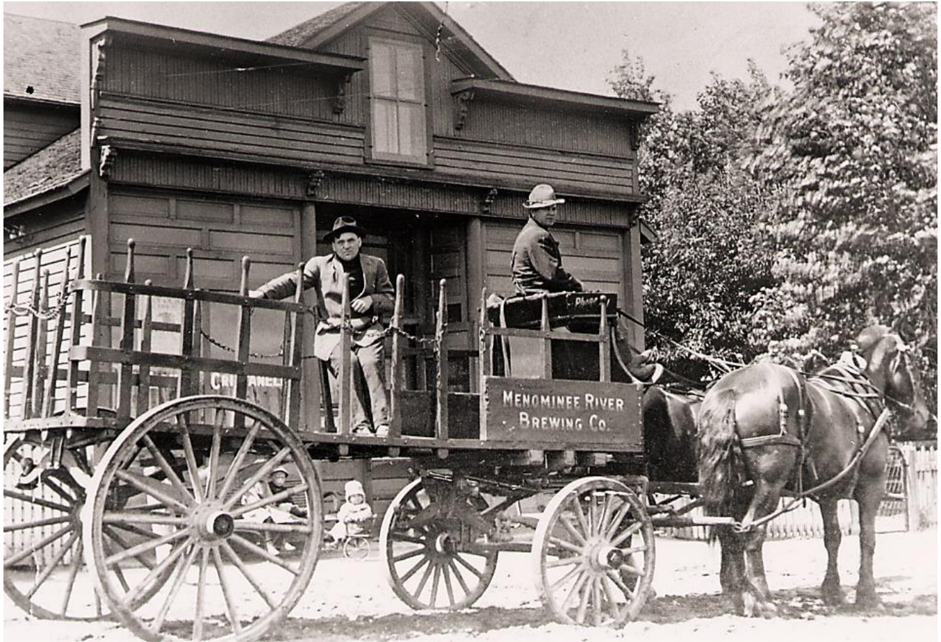
Louis Cristanelli's Saloon, 1009 Railroad Street, Norway, ca. 1914-1915: This postcard view taken in about 1914-1915 shows an empty Menominee River Brewing Company beer wagon in front of Louis Cristanelli's saloon at 1009 Railroad Street in Norway. Note the three children seated on the saloon steps behind the wagon wheels. [James Lindstrom]
