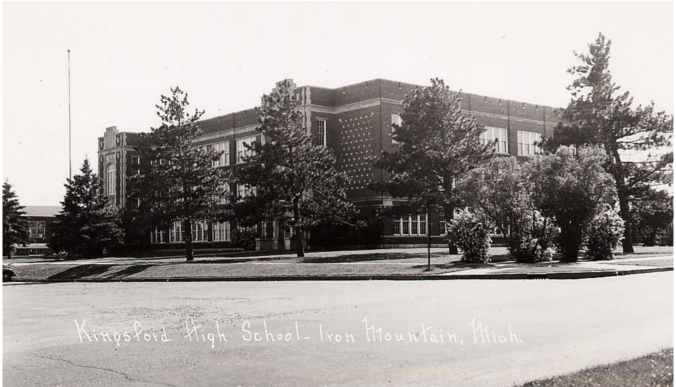
Kingsford High School, Hamilton Avenue, Ford Addition, Kingsford, ca. 1940-1950: This postcard view of Kingsford High School, taken from Hamilton Avenue and dating from 1940-1950, shows the east and north sides of Kingsford High School with the vocational building in the background to the left of the flagpole. The upper floor contained home economics and drafting classrooms, while shop classes were located on the lower level. [William John Cummings]
