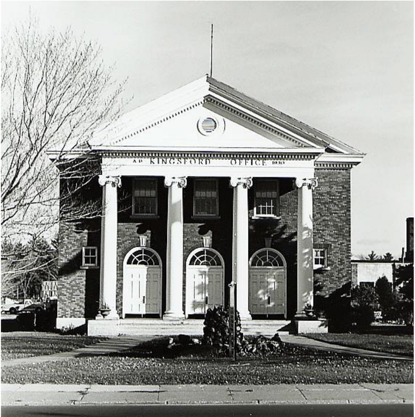
Kingsford City Hall, Southeast Corner of Carpenter Avenue and Hamilton Avenue, Kingsford, ca. 1940-1950: The Village of Kingsford began operations in its new office building on the southeast corner of the intersection of Carpenter Avenue and Hamilton Avenue on Monday, November 24, 1930. Prior to that time, village business was conducted in a couple of rooms in the basement of the Woodward Avenue School which were rented by the village at $10 per month. A village warehouse and garage were constructed in conjunction with the village hall. [City of Kingsford]
