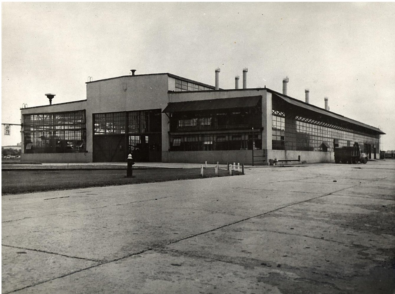
Ford Motor Company Maintenance Building "M", View from Southwest Corner, Kingsford, ca. xxxx: [Menominee Range Historical Museum]
