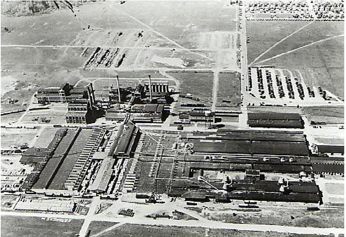
Ford Motor Company Plant in Kingsford, Looking North, ca. 1940-1950: This view of the Ford Motor Company's plant in Kingsford shows the complex and the southwest corner of the Ford Addition in the upper right corner. Note the parking lot just north of the plant in the Ford Field. [Jack Deo, Superior View Studio]
