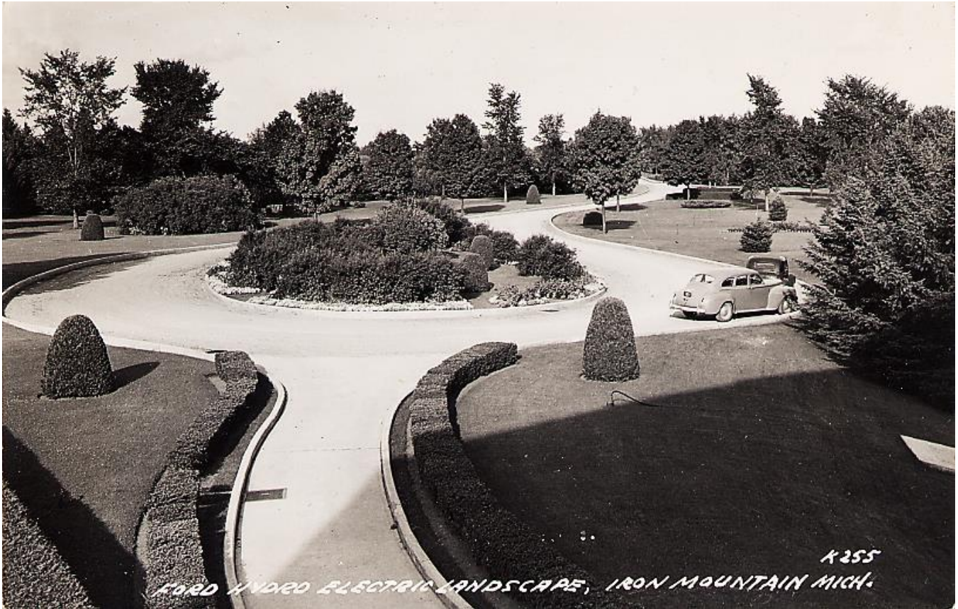
Ford Hydro-Electric Plant on the Menominee River, Kingsford, ca. 1940-1945: Taken from the doors leading into the power house, the landscaped grounds can be seen. At the far left the word "Ford" was planted in flowers to imitate the famed company logo on a berm. [William John Cummings]
