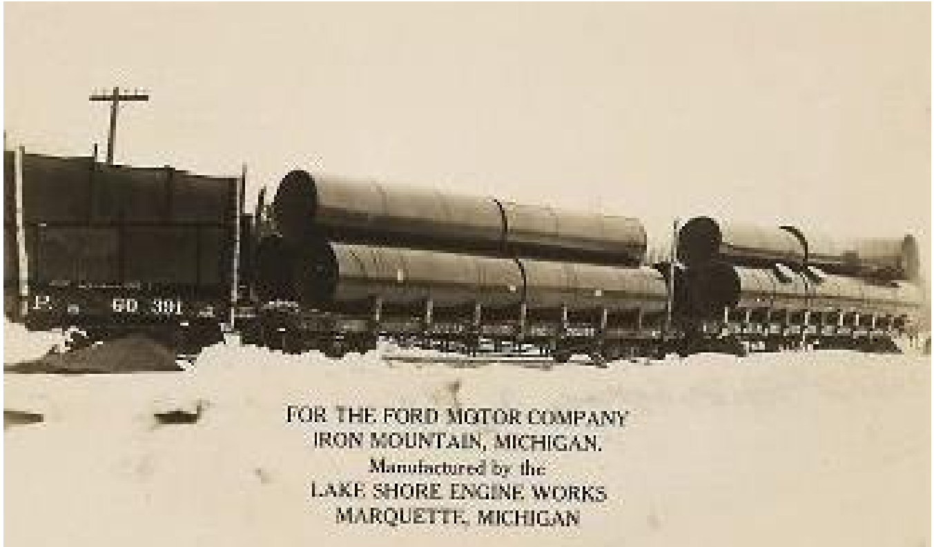
Ford Motor Company, Kingsford, ca. XXXX: This postcard view shows a shipment of horizontal flue pipe used at the Ford Motor Company's plant in Kingsford, manufactured by the Lake Shore Engine Works of Marquette, Michigan. [Guy Forstrom]
