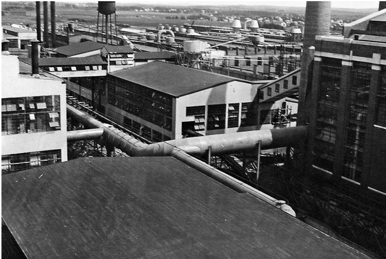
Saw Mill and Power House from the Rooftop of the Distillation Building, Ford Motor Company Plant, Kingsford, August, 1924: [Guy Forstrom]
