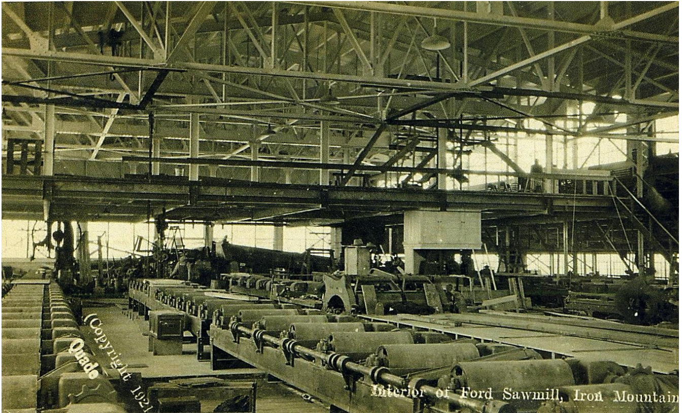
Interior of the Ford Motor Company's Saw Mill in Kingsford, 1921: Postmarked Iron Mountain, Mich., November 13, 1926, this Interior of Ford Sawmill, Iron Mountain, was taken by Albert Quade in 1921, possibly shortly after the sawmill opened in July. [William John Cummings]
