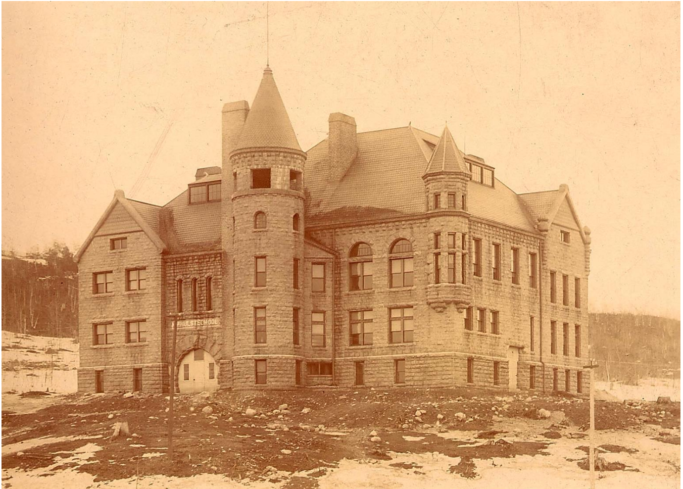
Nelson P. Hulst High School, Madison Avenue, Iron Mountain, ca. 1892: The school name, N.P. Hulst School, can clearly be read above the arched doorway with its temporary door, used during construction, still in place. The foundation was laid in 1891, and the school was completed in 1892, at about the time this photograph was taken. The school opened November 14, 1892. [Keen Scott]
