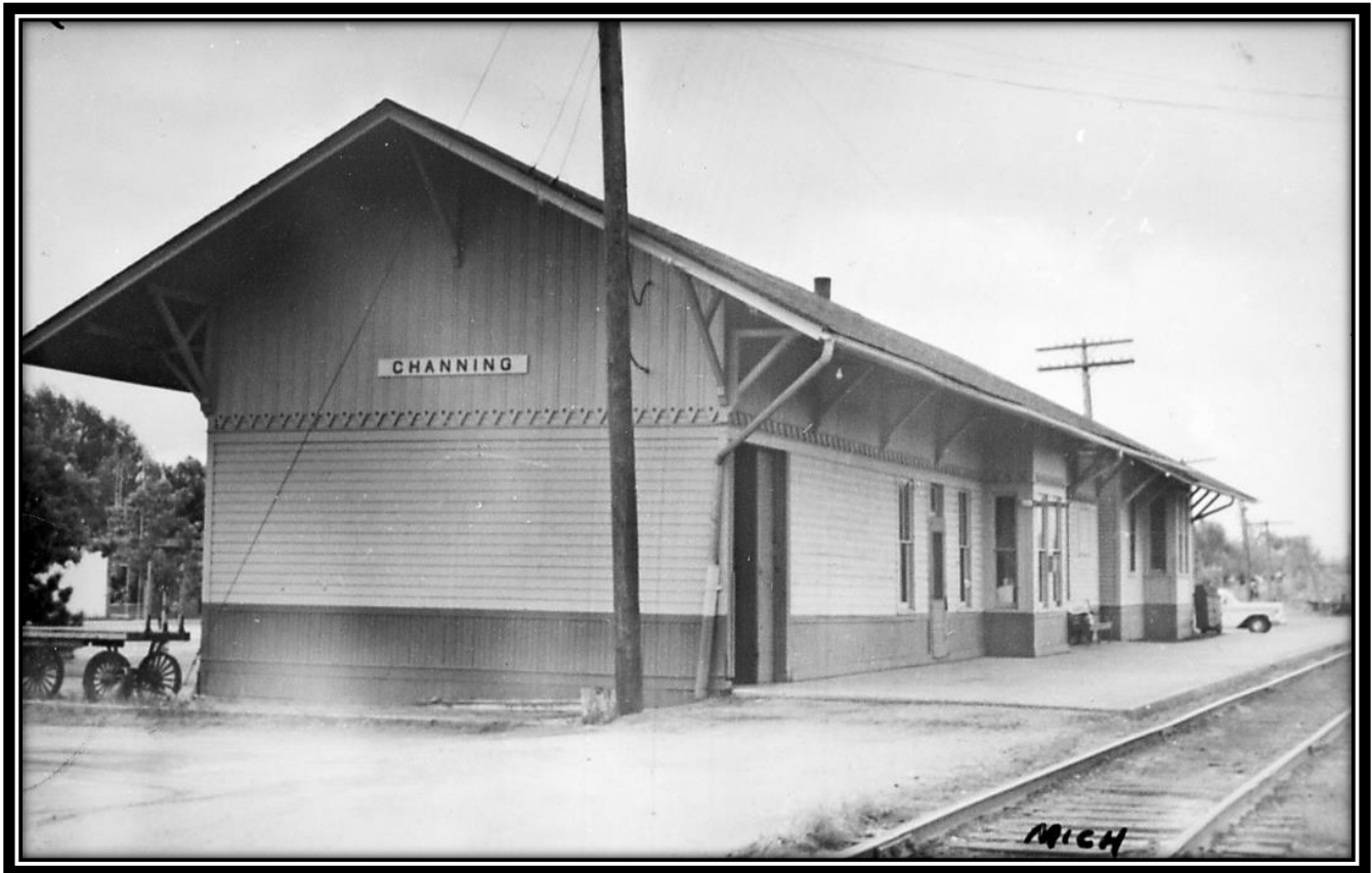
Chicago, Milwaukee & St. Paul Railway Depot, Channing, Dickinson County, Michigan, ca. 1950-1960: This unused real photo postcard view unidentified on the image shows the north end of the Chicago, Milwaukee & St. Paul Railway Depot with the tracks going southward on the west side of the building. This image was printed on Kodak paper and was reproduced from an original photograph. [William J. Cummings]
