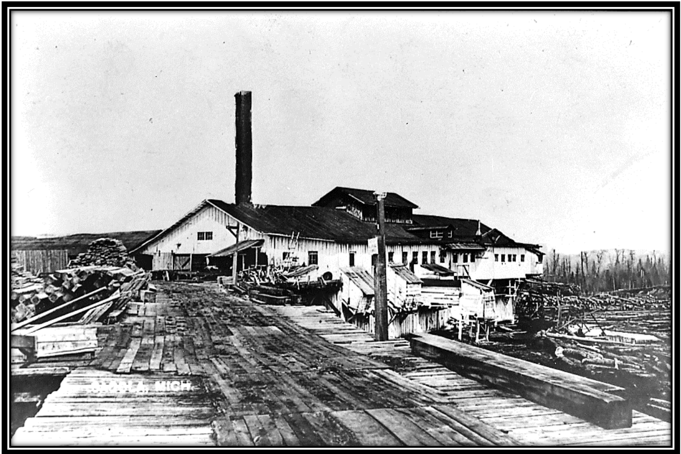
First Sagola Lumber Company Saw Mill, Sagola, ca. 1910: This postcard view of the first Sagola Lumber Company Saw Mill shows the wood plank tramway leading to the area where the lumber was stacked and stored. Note the millpond at the right. [Unknown Source]
