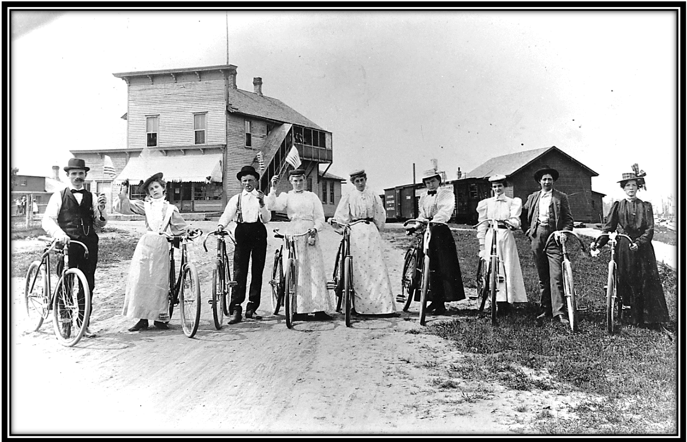
Bicyclists in Front of Sagola Lumber Company Store, July 4, 1905: Nine Sagola bicyclists dressed in their finest summer apparel posed in front of the Sagola Lumber Company Store on July 4, 1905. The store's warehouse can be seen in the background at the right. Mary Broadland, fourth from left, waved a flag over her head. Maude Wifler stood third from the right. Others said to be pictured here are Jacob Johnson, ----- Yuppenlotz, Hulda Wiberg, Louis Byers and ----- Price. [Ida Swanson]
