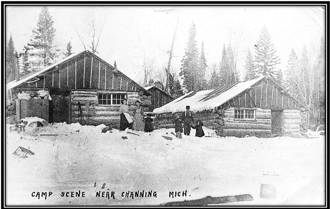
Logging Camp, Near Channing, ca. 1913: Postmarked Crystal Falls, Mich., in 1913 [day and month not visible on cancellation] , this camp scene appears to be an unidentified logging camp with the traditional log buildings with tarpaper gabled ends and roofs. Two women, a man and three children posed for the photographer. [William J. Cummings]
