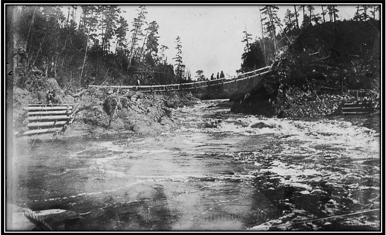
Swinging Bridge, Near Vulcan, Norway Township, Dickinson County, Michigan, ca. 1907: This real photo postcard view unidentified on the image shows the Swinging Bridge near Vulcan and is postmarked Vulcan, Michigan, April 6, 1907. Note the people walking across the bridge. [William J. Cummings]
