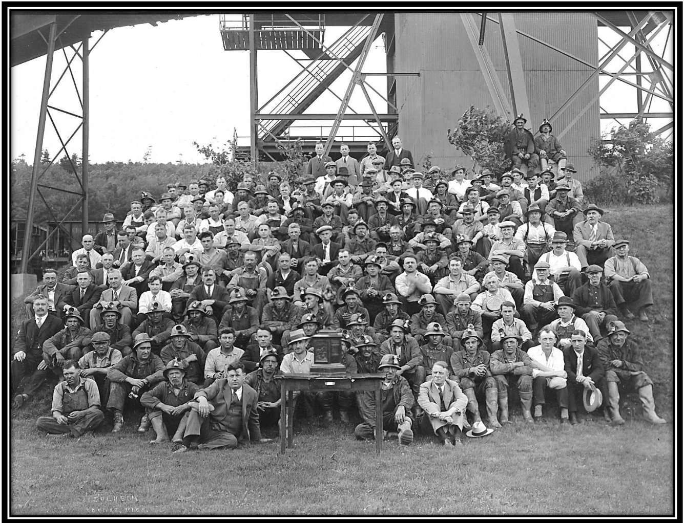
East Vulcan Mine Safety Award, East Vulcan Mine, Vulcan, Dickinson County, Michigan, July 1931: These miners and other employees posed for the presentation of the Vulcan Mine Safety Award in July 1931. The statue on the table represents St. Barbara, the patron saint of miners. Saint Barbara is venerated by Catholics who face the danger of sudden and violent death at work. She is the patron of miners, tunnellers, armorers, military engineers, gunsmiths and anyone else who worked with cannon and explosives. Note the embossed “Solheim, Norway, Mich.” identification at the lower left. This photograph appears on page 37 in Vulcan, Michigan, Centennial Book 1872-1972 . [Menominee Range Historical Museum]
