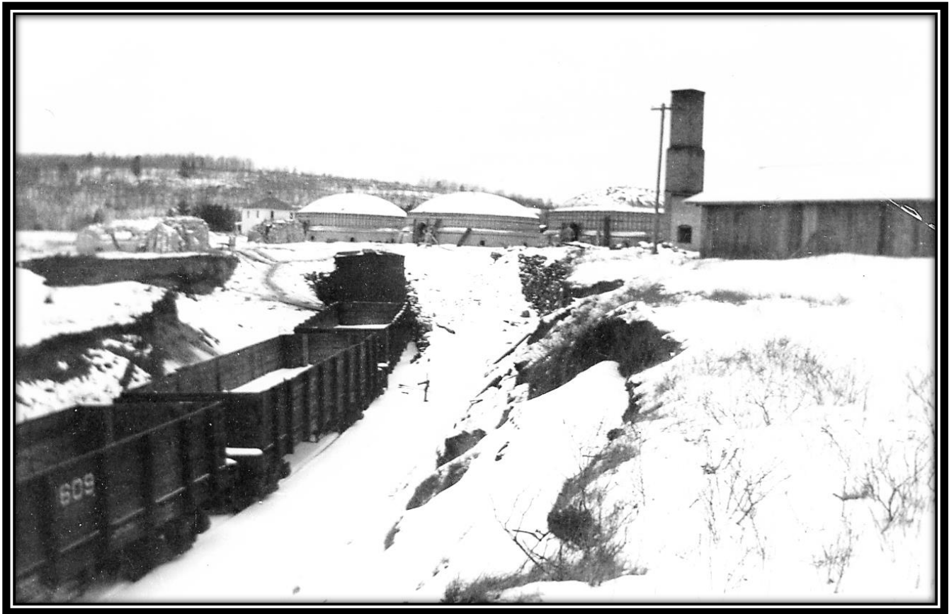
Vulcan Brick Works, Near Vulcan, Dickinson County, Michigan, ca. 1925: Dating to about 1925, this photograph of the Vulcan Brick Works shows the railroad siding, the three brick kilns and various buildings, including the superintendent's house in the background to the left of the kilns. Beginning in the winter of 1932, Noel H. Turner began producing local peat which was briquetted and used as fuel particularly well-suited for burning clay ware such as bricks. This photograph appears on page 59 in Vulcan, Michigan, Centennial Book 1872-1972 . [Menominee Range Historical Museum]
