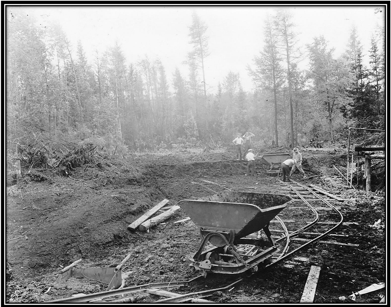
Vulcan Brick Works, Near Vulcan, Dickinson County, Michigan, ca. 1910-1915: Dating between 1910 and 1915, dump cars were being loaded with clay at the Vulcan Brick Works. [Menominee Range Historical Museum]
