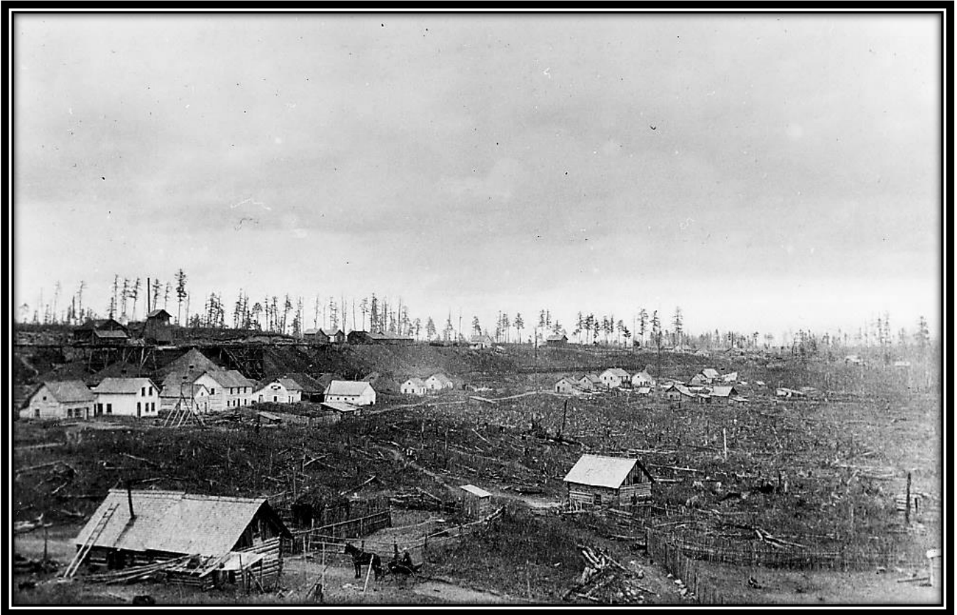
East Vulcan Mine Looking Northeast, East Vulcan, Menominee County (later Dickinson County), Michigan, May 1886: Taken in May 1886, this view, looking northeast, shows the East Vulcan Mine, located on the S \frac{1}{2} of the S \frac{1}{2} of Section 11, T39N, R29W. A shaft house appears above the tramways and stockpiles in the upper left. Notice how the land has been clear-cut with few trees remaining on the horizon. This photograph appears on page 35 in Vulcan, Michigan, Centennial Book 1872-1972 . [Marquette County Historical Society]
