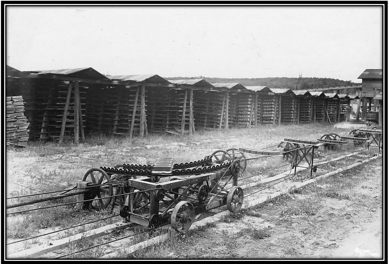
Vulcan Brick Works, Near Vulcan, Dickinson County, Michigan, ca. 1925: In 1924, Noel H. Turner, a son of William J. Turner, reopened and rebuilt the brick plant, moving the entire operation to a higher location about a quarter of a mile east of the original site. Dating from about 1925, this view of the Vulcan Brick Works shows the drying sheds with stacks of bricks and conveyors on tracks used for transporting them. This photograph appears on page 59 in Vulcan, Michigan, Centennial Book 1872-1972 . [Menominee Range Historical Museum]
