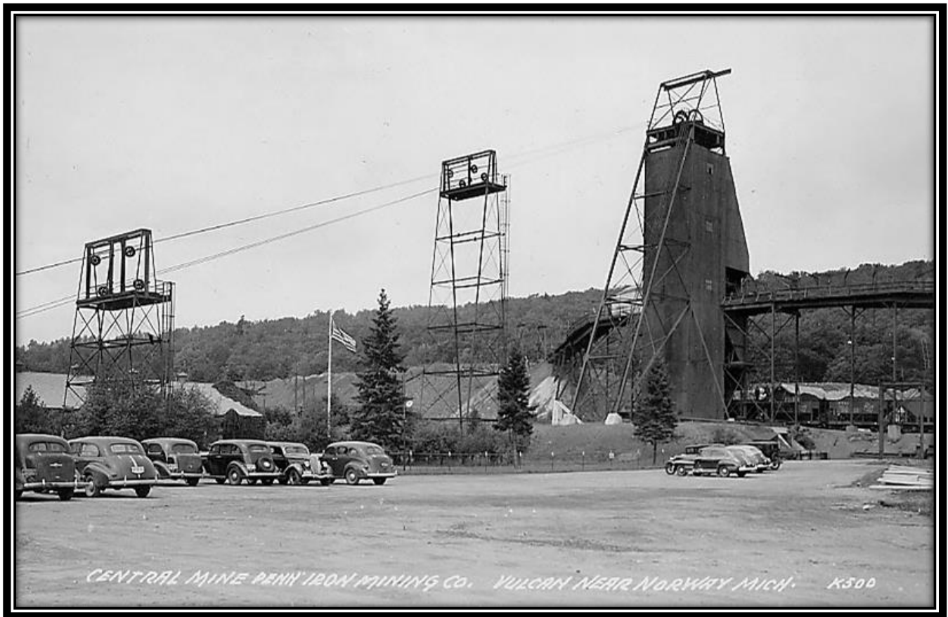
Central Vulcan Mine, Penn Iron Mining Company, Vulcan, Dickinson County, Michigan, ca. 1939-1945: This unused real photo postcard view identified as the "Central Mine, Penn Iron Mining Co., Vulcan, Near Norway, Mich. K500" dates from between 1939 and 1945 with an EKC stamp box to indicate its age. Note the cars in the parking lot. [William J. Cummings]
