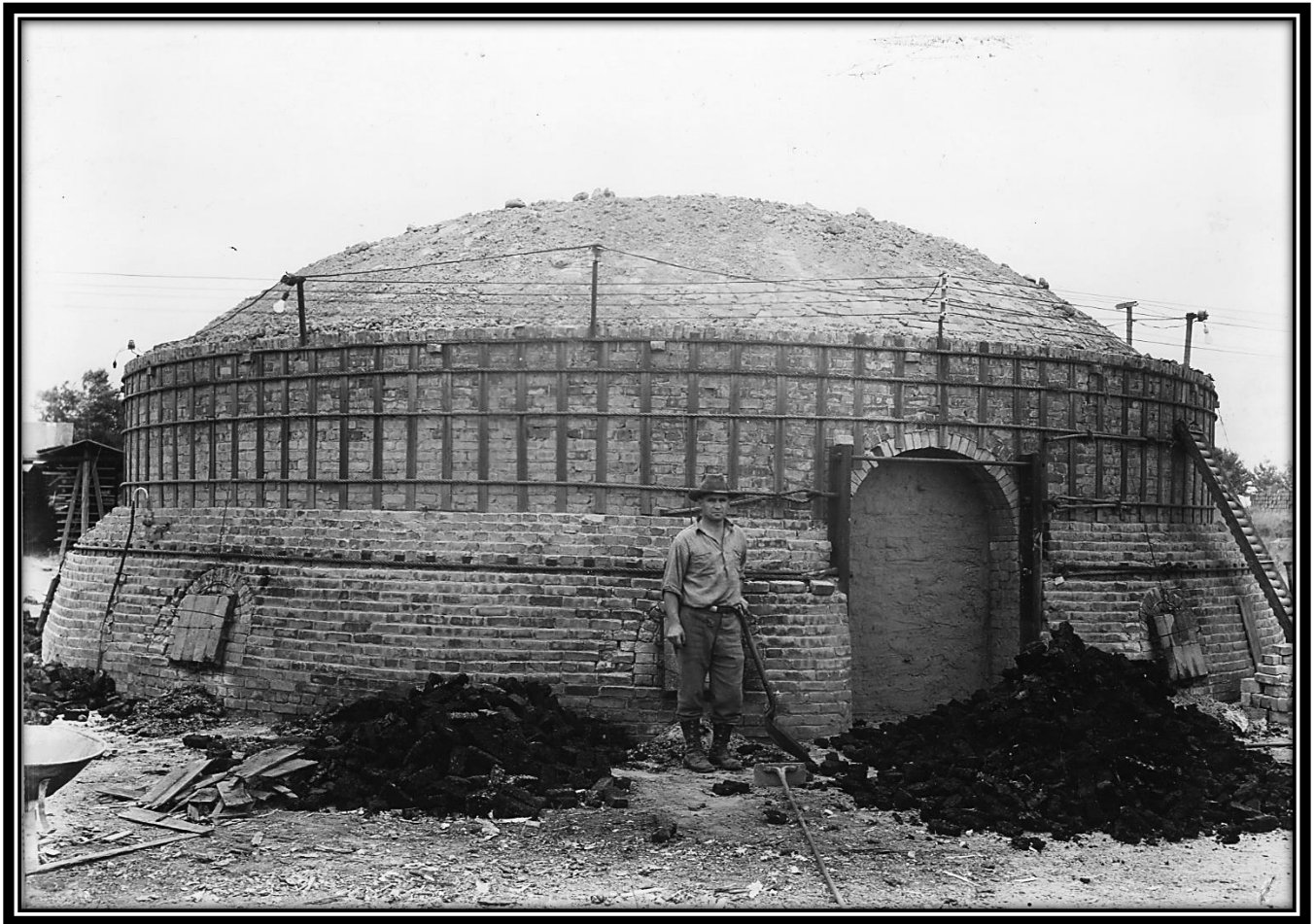
Vulcan Brick Works, Near Vulcan, Dickinson County, Michigan, ca. 1925: The wood-burning “scove kilns” were replaced by more efficient coal fired “Boss kilns” with forced and induced draft equipment. Dating from about 1925, a worker stood next to one of the kilns at the Vulcan Brick Works. Note the charcoal piles and the construction of the kiln. [ Menominee Range Historical Museum ]
