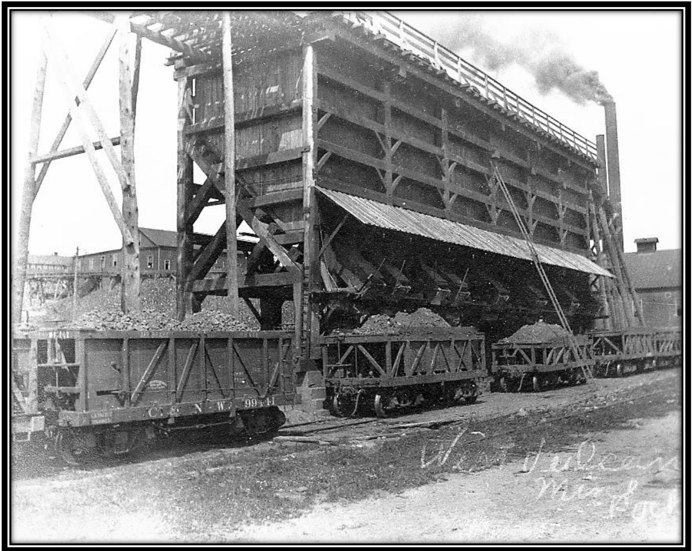
West Vulcan Mine, Vulcan, Dickinson County, Michigan, ca. 1910-1915: This unused real photo postcard view identified as the "West Vulcan Mine" probably dates between 1910 and 1915 and shows the loading process used at the mine from the tramway. Note the loading chutes and the five railroad ore cars, three of which are loaded. [William J. Cummings]
