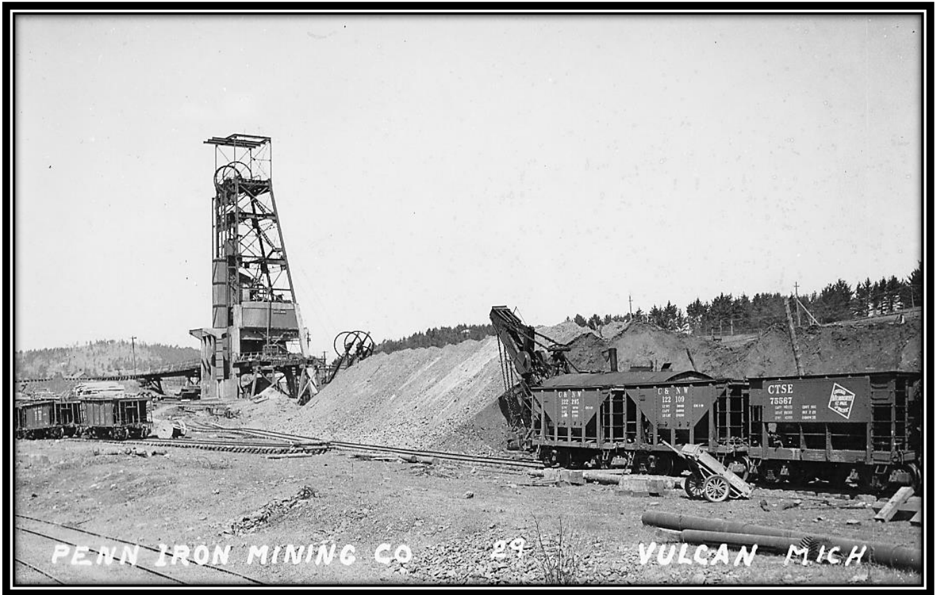
Central Vulcan Mine, Penn Iron Mining Company, Vulcan, Dickinson County, Michigan, ca. 1925-1942: This unused real photo postcard view identified as “ Penn Iron Mining Co. 29 Vulcan, Mich. ” probably dates between 1925 and 1942 with a DOPS stamp box to indicate its age. The mine shaft at the left might be the Curry Shaft. The steam shovel in the center was used to fill the ore cars which are seen on the railroad tracks on both sides of this photograph. [William J. Cummings]
