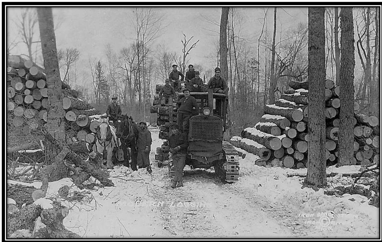
Steam Hauler, Unidentified Logging Operation, Iron River, Iron County, Michigan, ca. 1925-1942: This unused real photo postcard view identified as “Modern Logging” probably dates between 1920 and 1925 and was published by the Iron Range Studio, Iron River, Michigan. A steam hauler is shown on the logging road, as well as a team of horses at the left. [William J. Cummings]
