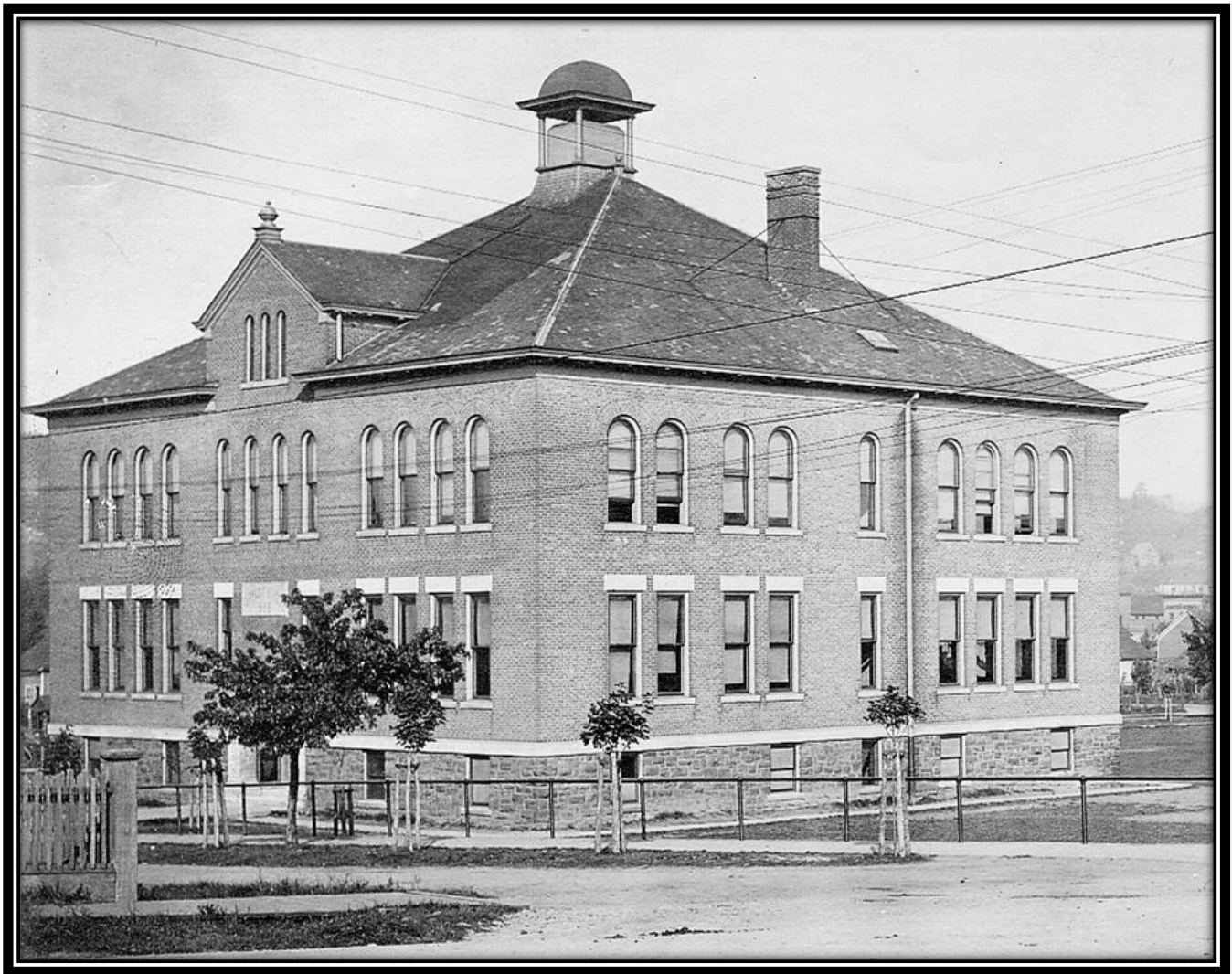
Farragut School, Corner of Vulcan Street and Fifth Street, North Side, Iron Mountain, Dickinson County, Michigan, October 19, 1912: Located at the corner of Vulcan and Fifth Streets in the Chapin Location (North Side), this view of the Farragut School is dated October 19, 1912. Constructed in 1899, the two-story brick structure, named in honor of Admiral David Glasgow Farragut, admiral of the U.S. Navy during the Civil War, best remembered in popular culture for his order at the Battle of Mobile Bay, usually paraphrased “Damn the torpedoes, full speed ahead.” [Menominee Range Historical Museum]
