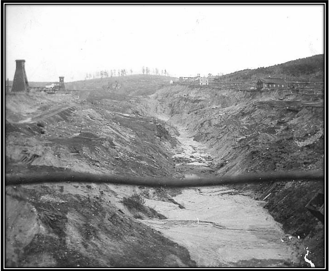
Chapin Mine Cave, East Side of the Chapin Pit, Chapin Location, North Side, Iron Mountain, Dickinson County, Michigan, 1899: This photograph documents the gradual settling of ground around the Chapin Mine into what is now known as the Chapin Pit. The camera is facing northeast and some of the earliest Chapin Mine shaft houses are visible at the left. The buildings just right of center in the distance are probably a part of the Millie Mine. The dark-colored building at the right in the distance is probably a part of the Chapin Mine complex. [Keen Scott]
