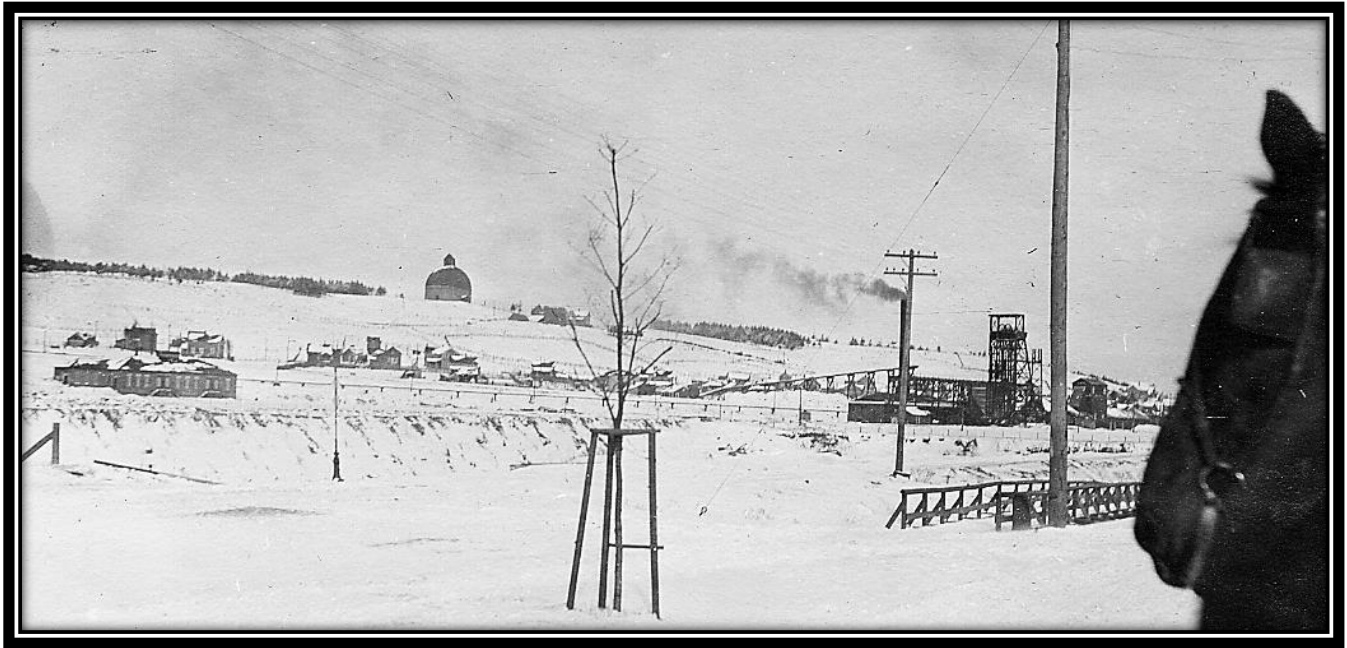
Hamilton Mine Shaft, Chapin Location, North Side, Iron Mountain, Dickinson County, Michigan, ca. 1913: This view of the Hamilton Mine Shaft at the right was taken in about 1913 by an amateur photographer. The head of the photographer's horse appears at the extreme right. The round sandstone water tank with its cast iron dome can be seen left of center on the horizon. [Menominee Range Historical Museum]
