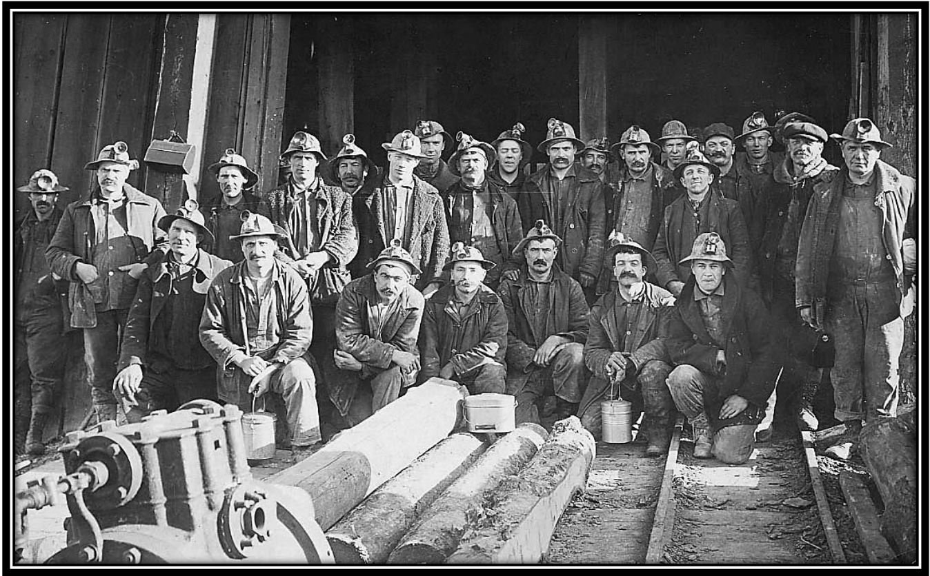
Unidentified Group of 25 Miners in Front of Shaft House , (showing group of twenty-five miners in front of shaft house with skip entrances behind them and logs being made into timbers in front; men wearing carbide lamps on their hats and three kneeling miners have round or oval lunchpails; tracks leading to skip shaft and cage for miners to the left of this shaft; acquired in Dickinson County by seller), unused (real photo, AZO Stamp Box with Four Triangles Up, ca. 1904-1918) [2010 – Jim Stearns, Iron Mountain, MI -- $9.10] $20.00 [William J. Cummings]
