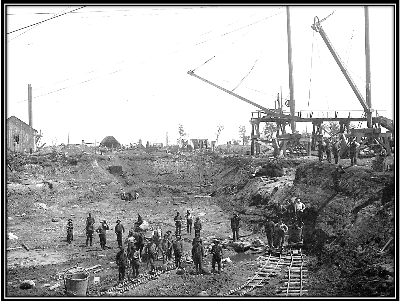
Florence Mine, Florence, Florence County, Wisconsin, 1890: Taken by Jorgen Johansen Eskil, pioneer Menominee Range photographer who operated his studio in Florence beginning on July 4, 1883 and moved to Iron Mountain in 1891, this view, dating from 1890, probably shows the Florence Mine. Note the men working in the open pit with temporary railroad tracks and the large ore bucket at the lower left. There is a possibility that this could also be the Badger Mine. [Menominee Range Historical Museum]
