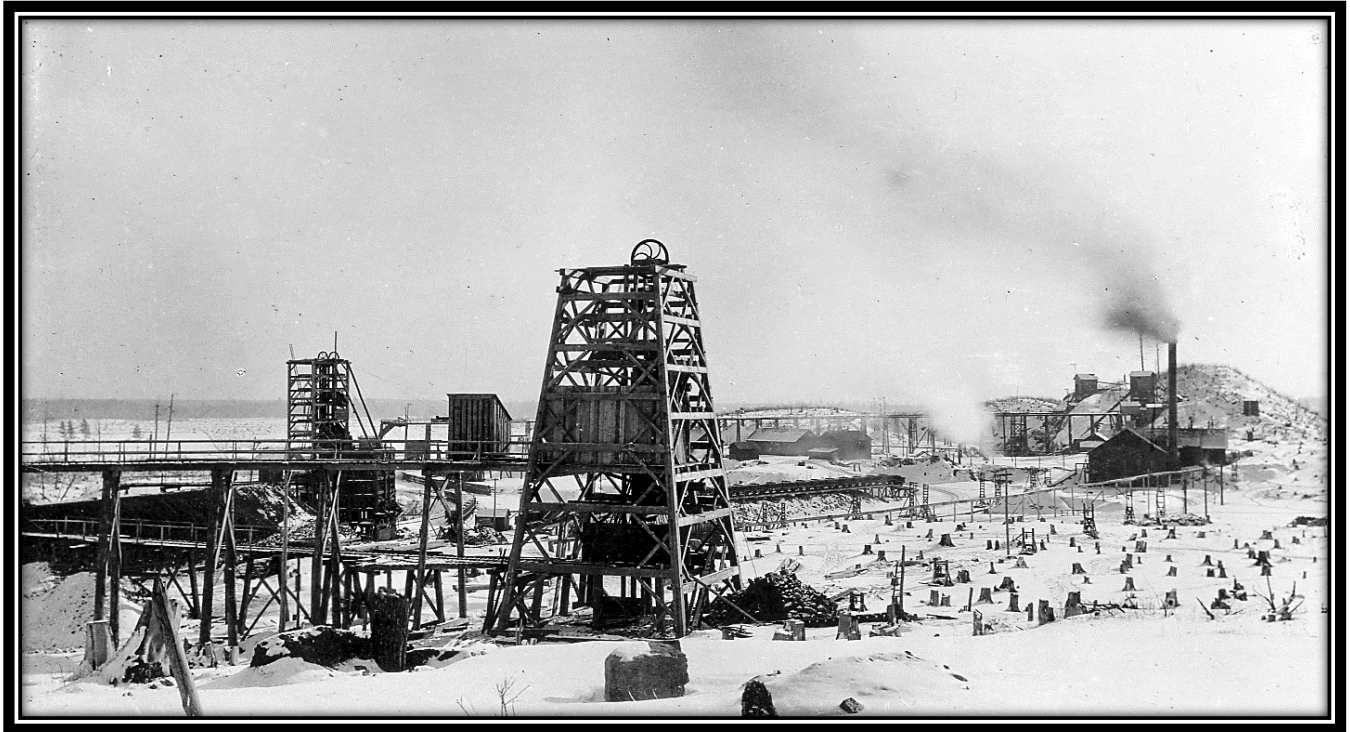
Florence Mine, Florence, Florence County, Wisconsin, 1890: Taken by Jorgen Johansen Eskil, pioneer Menominee Range photographer who operated his studio in Florence beginning on July 4, 1883 and moved to Iron Mountain in 1891, this view, dating from 1890, shows the Florence Mine. Note the wooden shaft housing in the center, the various tramways and trestles and various mining buildings in the distance. [Menominee Range Historical Museum]
