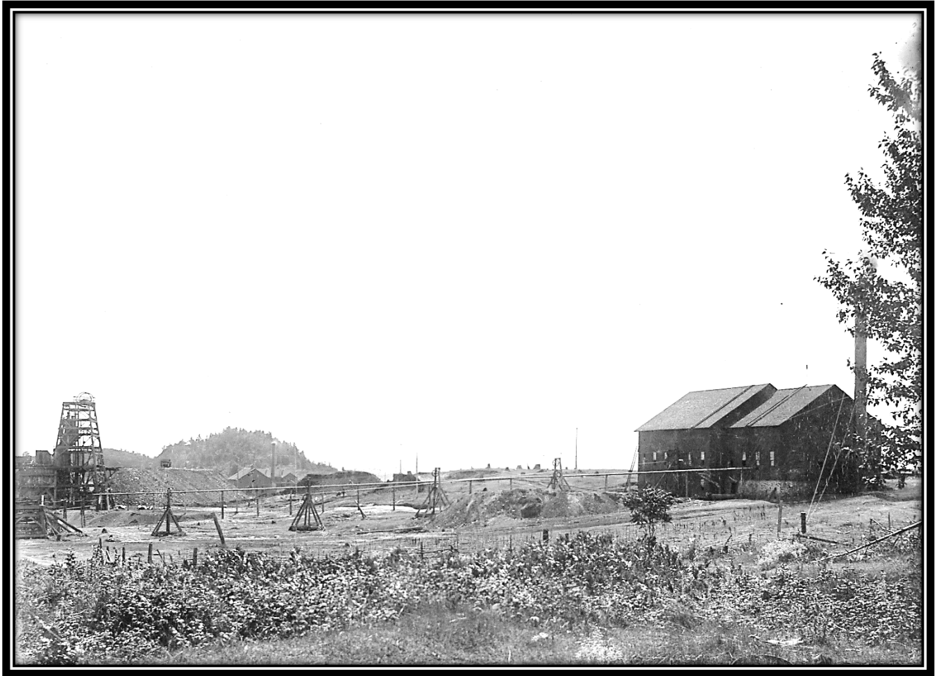
Florence Mine, Florence, Florence County, Wisconsin, 1886: Taken taken by Jorgen Johansen Eskil, pioneer Menominee Range photographer who operated his studio in Florence beginning on July 4, 1883 and moved to Iron Mountain in 1891, this view, dating from 1886, shows the Florence Mine. Note the wooden shaft housing at the far left. [ Menominee Range Historical Museum ]
