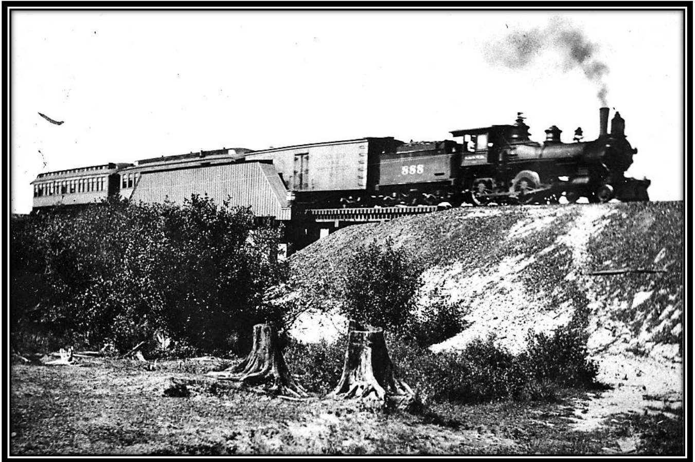
The Felch Flyer, Foster City, Felch Township, Dickinson County, Michigan, August 1910: This real photo postcard view unidentified on the image caught “The Felch Flyer,” also called “The Lightning Express,” crossing the railroad bridge over the Sturgeon River at Foster City in August 1910. Note the two passenger cars behind the boxcar. [Beatrice Blomquist]
