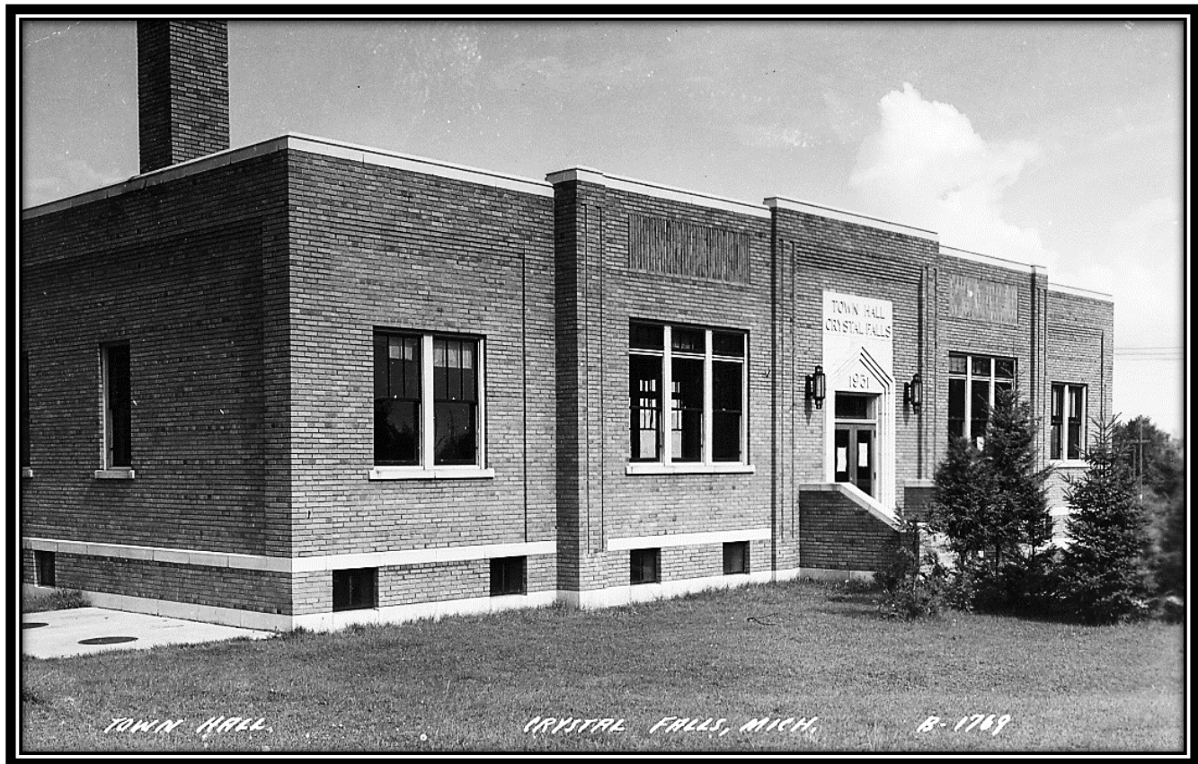
Crystal Falls Town Hall, 1384 U.S. 141, Crystal Falls, Iron County, Michigan, ca. 1940-1950: This unused real photo postcard view is identified as "Town Hall, Crystal Falls, Mich. B-1769." The Crystal Falls Town Hall was constructed in 1931 and is located at 1384 U.S. 141 in Iron County, Michigan. [William J. Cummings]
