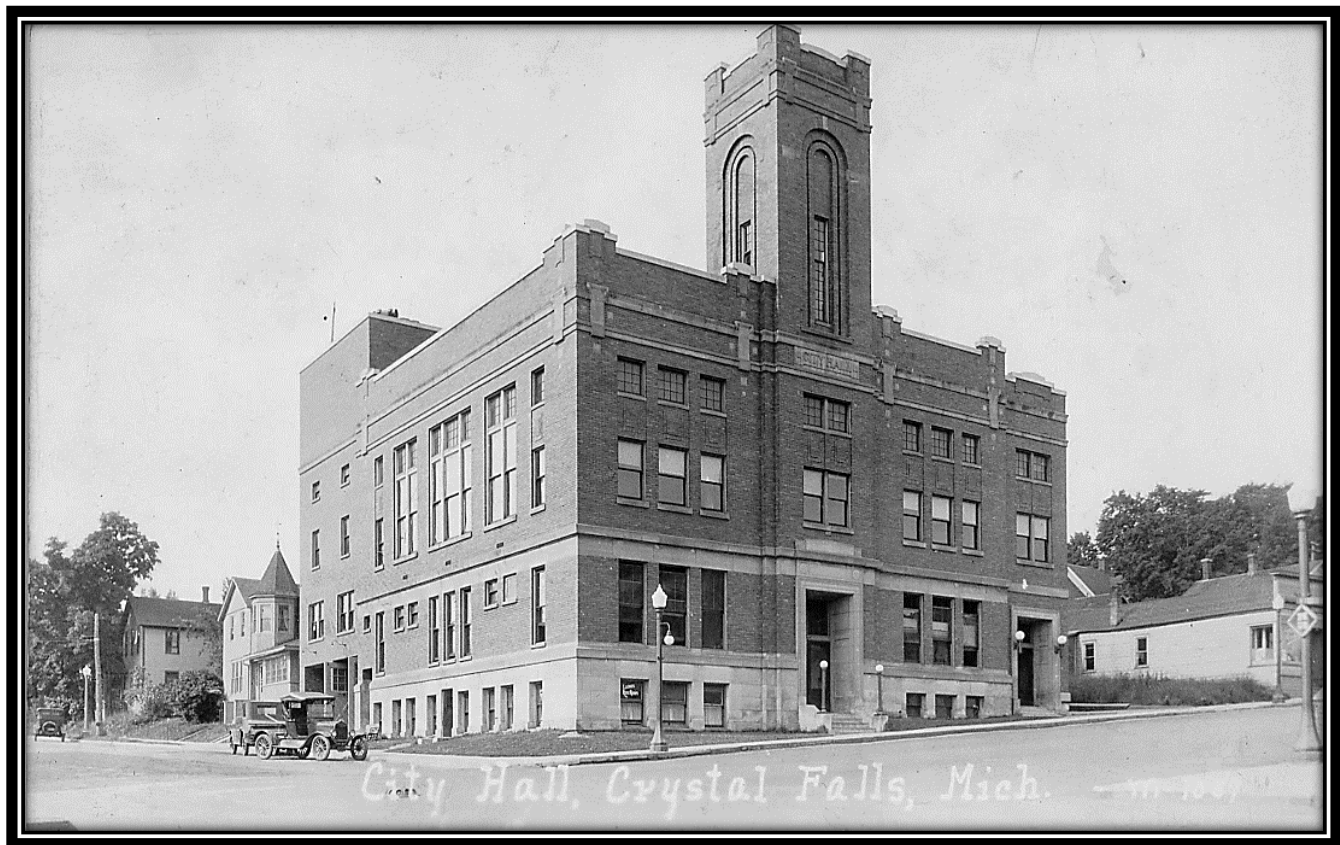
Crystal Falls City Hall, Superior Avenue, Crystal Falls, Iron County, Michigan, ca. 1930: This real photo postcard view identified as "City Hall, Crystal Falls, Mich." shows the Crystal Falls City Hall on the south side of Superior Avenue. Note the two old cars on the side of the building and the garage doors which served the fire department. [William J. Cummings]
