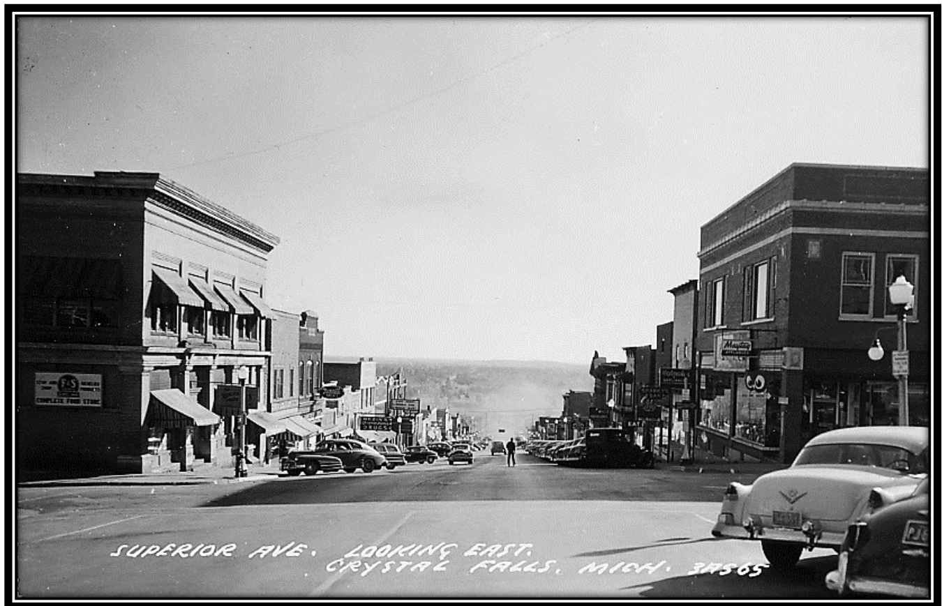
Superior Avenue, Looking East, Crystal Falls, Iron County, Michigan, ca. 1940-1950: This unused real photo postcard view identified as "Superior Ave. Looking East, Crystal Falls, Mich., 3N565" was at the U.S. 2 intersection, looking east, and shows the Finnish & Swedish (F. & S.) Mercantile Association store, the two-story brick building at the left, built in 1906. The sign for Rezin's Walgreen Agency Drugs can be identified midway down the north (left) side of the street. [William J. Cummings]
