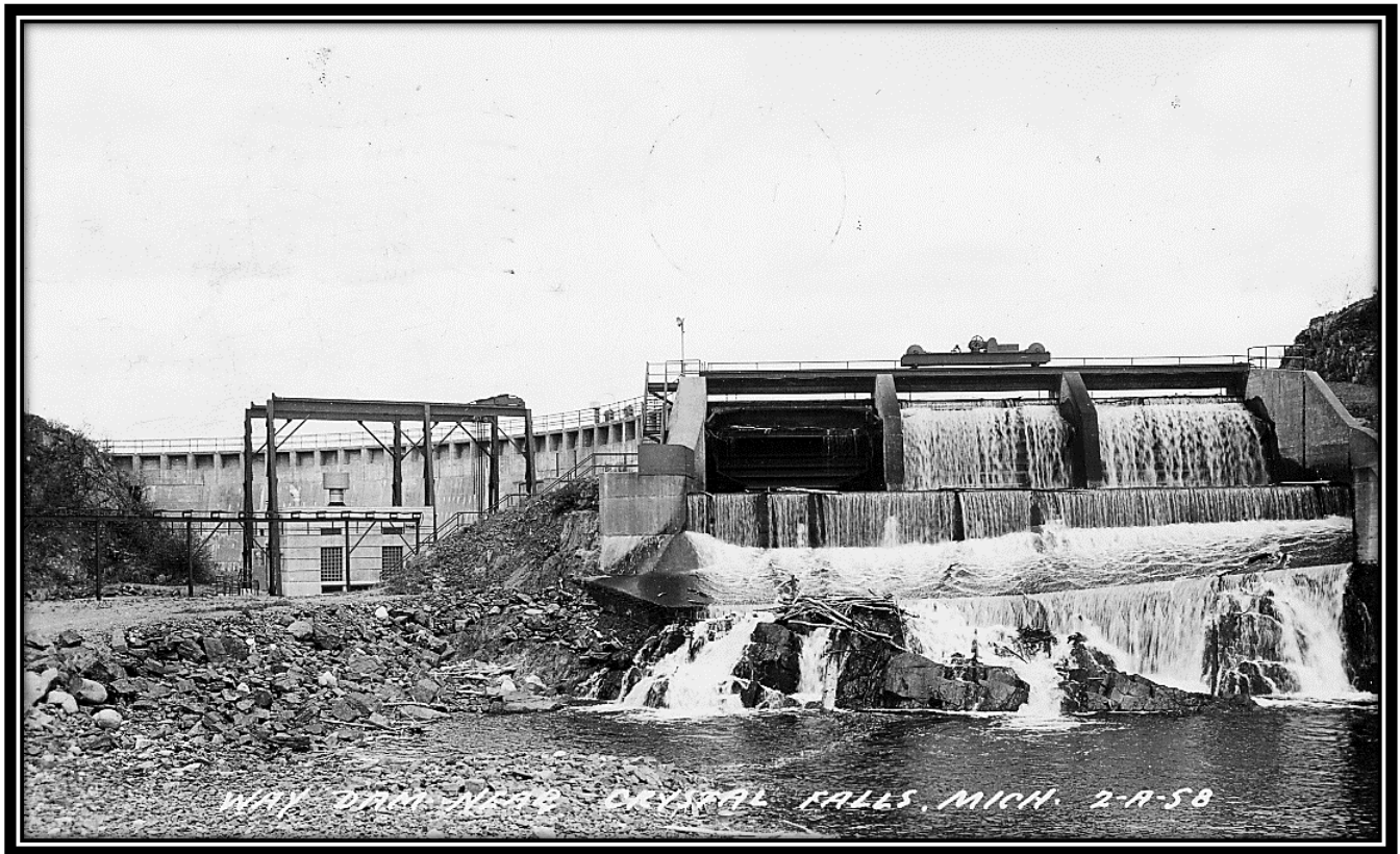
Way Dam, Near Crystal Falls, Iron County, Michigan, ca. 1961: This real photo postcard view identified as “Way Dam Near Crystal Falls, Mich. 2-A-58” and postmarked Crystal Falls, Michigan, October 11, 1961, shows Way Dam, located 6.3 miles east of Crystal Falls in Mansfield Township on the Michigamme River. The dam structure shows water cascading over two of the three dam gates with waterfalls below. [William J. Cummings]
