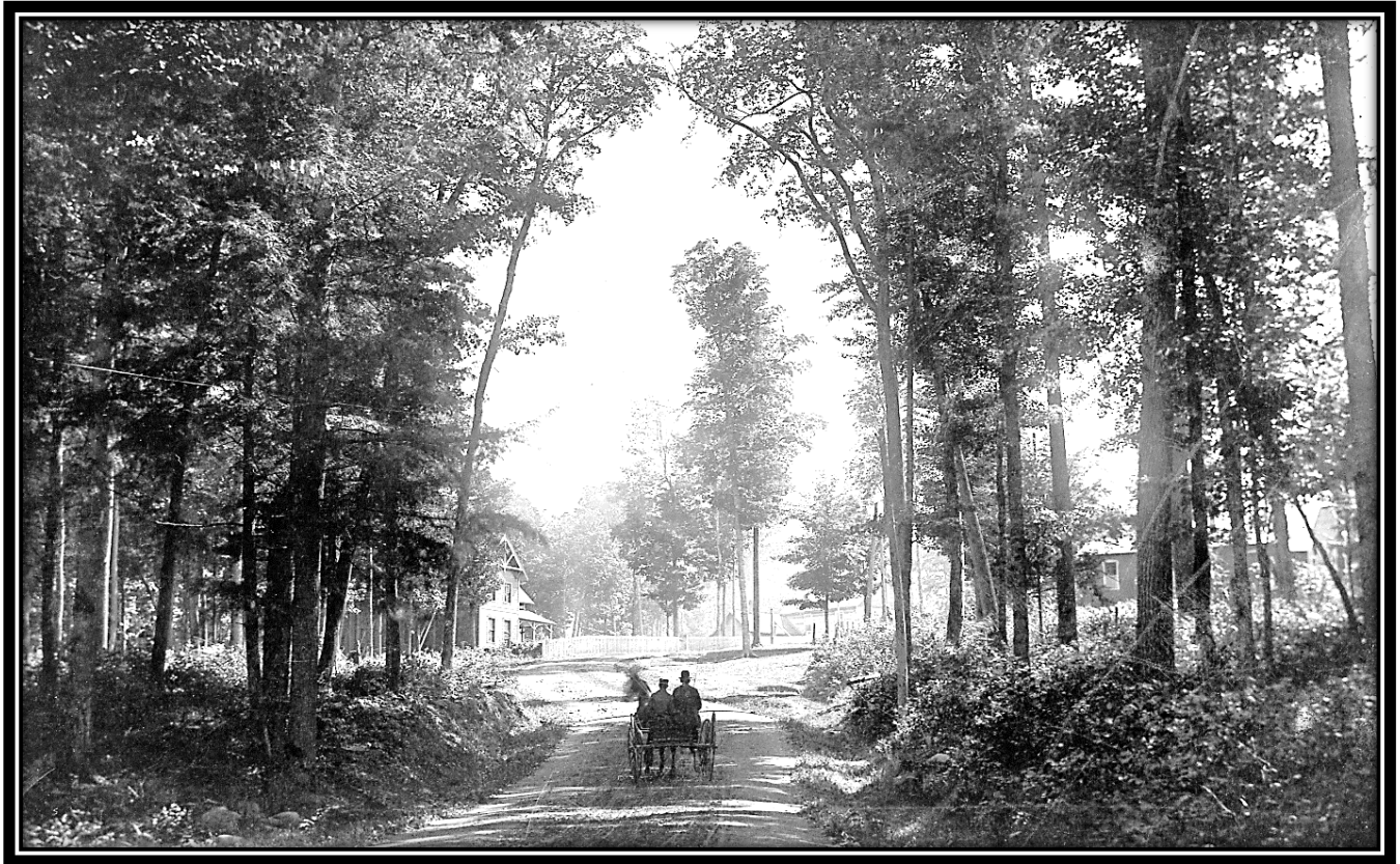
Road to the Commonwealth Mine with Superintendent's House and Office Buildings, Commonwealth, Florence County, Wisconsin, ca. 1890: Taken in about 1890 by Jorgen Johansen Eskil, pioneer Menominee Iron Range photographer, this view shows the road leading to the Commonwealth Mine with the superintendent's house at the left and office buildings to the right. [Menominee Range Historical Museum]
