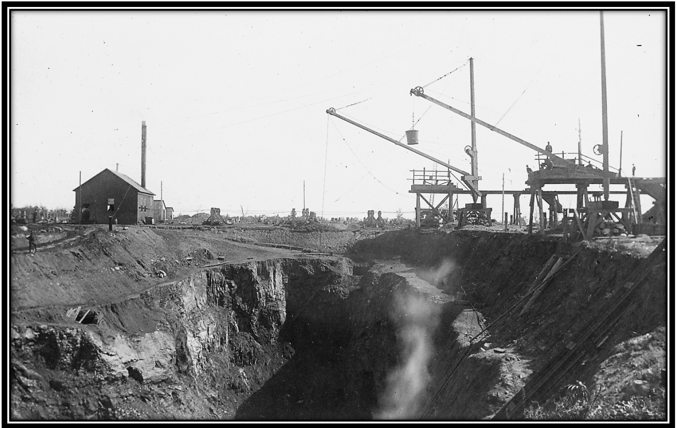
Badger Mine (or possibly the Florence Mine), Commonwealth, Florence County, Wisconsin, ca. 1890: Taken in about 1890 by Jorgen Johansen Eskil, an early photographer on the Menominee Iron Range with a studio in Florence, this view shows the Badger Mine. Another identical photograph is identified as the Florence Mine. Note the open pit and the huge bucket suspended from one of the timbers at the right. [Menominee Range Historical Museum]
