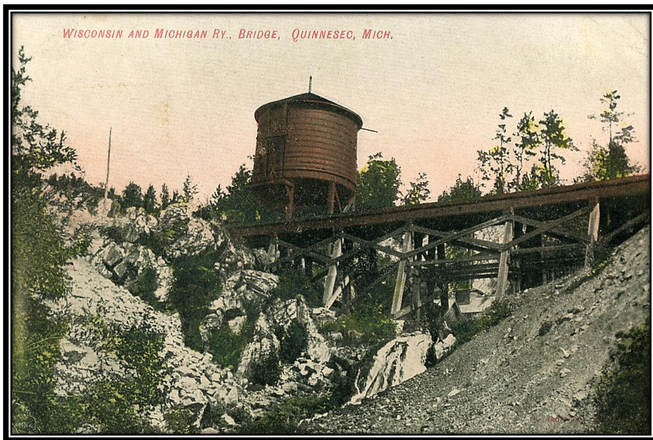
Wisconsin & Michigan Railway Bridge, Fumee Falls, East of Quinnesec, Breitung Township, Dickinson County, Michigan, ca. 1910-1915: This unused tinted black-and-white postcard view identified as the "Wisconsin & Michigan Ry. Bridge, Quinnesec, Mich." probably dates between 1910 and 1915. Note the huge water tank used to fill steam engine holding tanks. This site, just east of Quinnesec, was later developed into a tourist park and camp site. [William J. Cummings]
