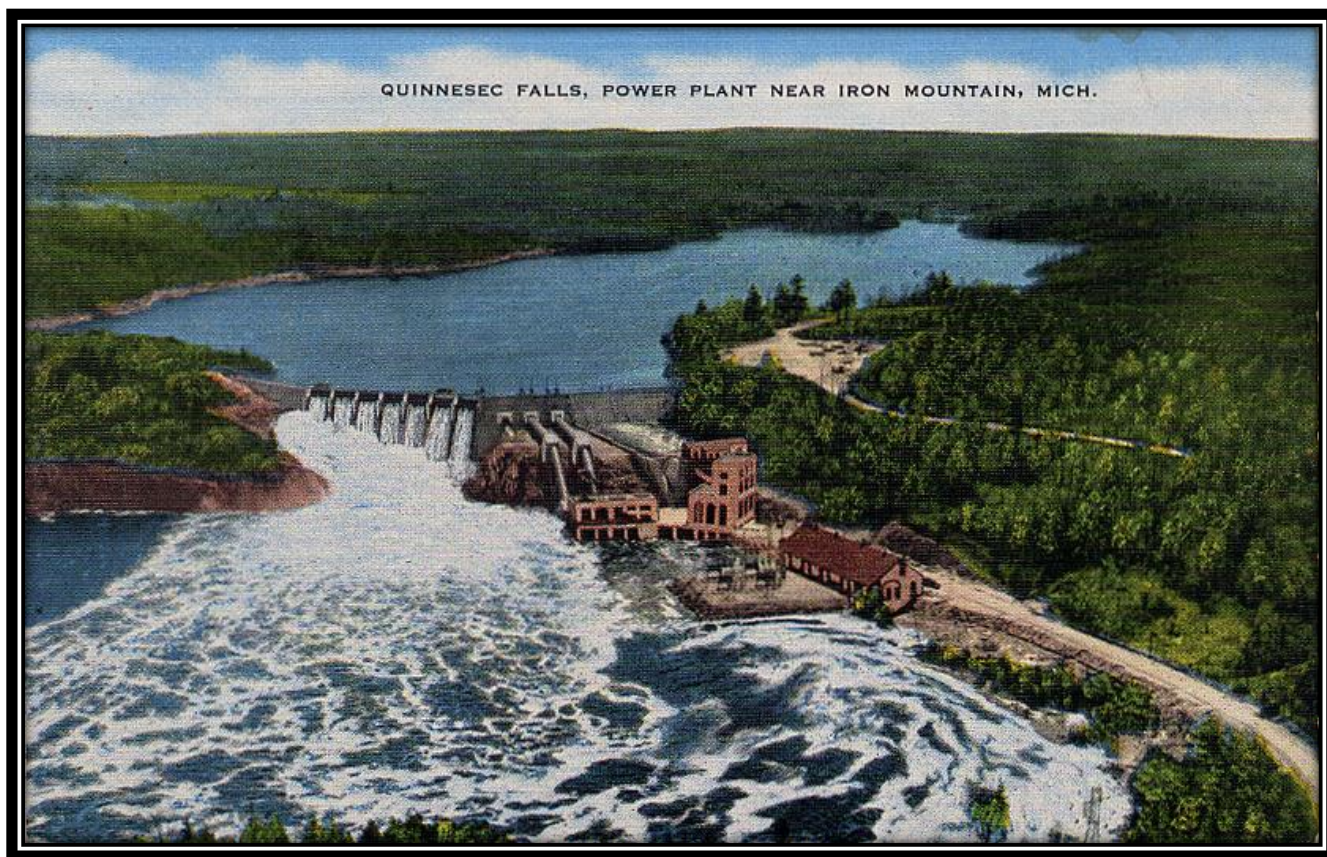
Hydraulic Falls (Upper Quinnesec Falls) Power Plant, Near Quinnesec, Breitung Township, Dickinson County, Michigan, ca. 1950: This colored black-and-white halftone postcard view identified as “ Quinnesec Falls, Power Plant Near Iron Mountain, Mich. ” probably dates from about 1950 and shows an aerial view of the Quinnesec Power Plant Complex. [William J. Cummings]
