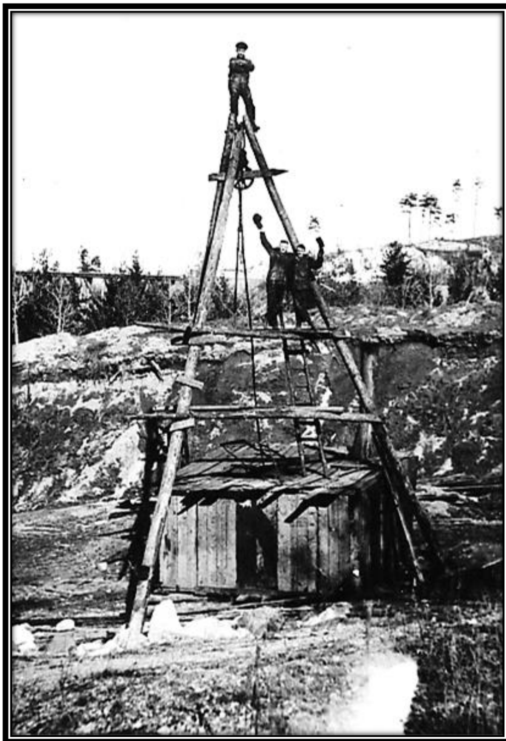
Diamond Drilling Operation, Near Fumee Creek on the McKenna Property, Quinnesec, Breitung Township, Dickinson County, Michigan, ca. 1910-1915: Walter Alquist, Axel Alquist and Amil LaPointe stood on the diamond drill scaffold, waving to the photographer. Note the Chicago, Milwaukee & St. Paul Railway bridge in the background at the left. [Roxanne Anderson]
