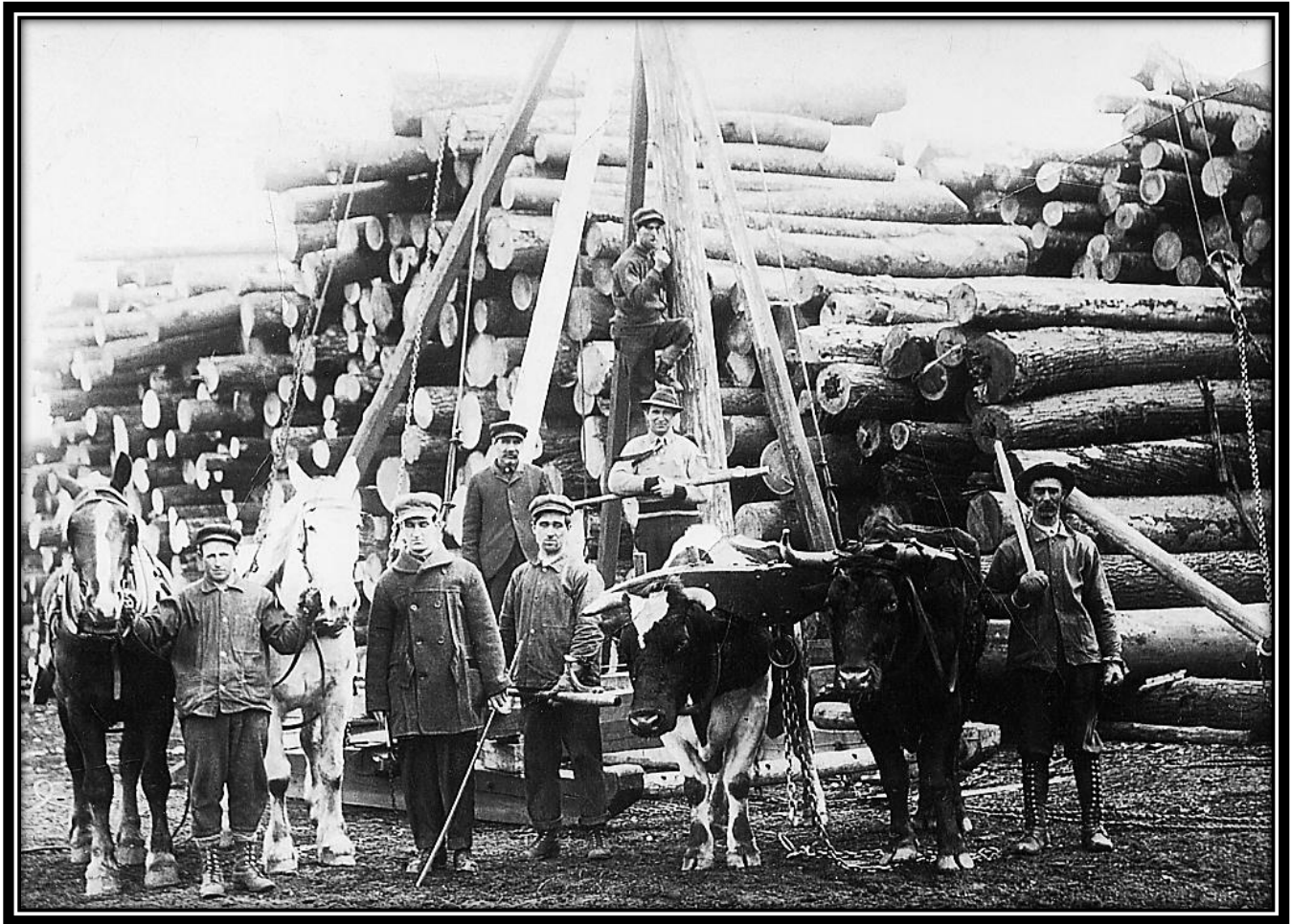
Decked Logs and Decking Crew, Near Foster City, Dickinson County, Michigan, ca. 1910-1915: This unused real photo postcard view with unidentified image probably dates between 1910 and 1915. A team of horses, held by their teamster, and a yoke of oxen provided power as logs were decked with this swing boom jammer. The man with the long prod was the driver in charge of the oxen. Unlike horses, oxen never became excited or panicked. Oxen required less care, lived on less feed and were seldom subject to illness or accident. Their equipment was simple and inexpensive. However, they moved at a provokingly slow gait. This postcard view was taken near Schaffer in Delta County, and La Branche in Menominee County, southeast of Foster City. [William J. Cummings]
