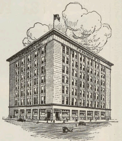
Patrick Company's general office and wholesale house
