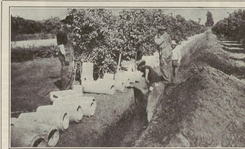
Draining a young orchard to lower ground water level
