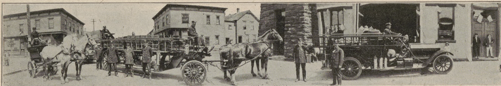
The up-to-date Fire Department of Ironwood, Clover-Land
