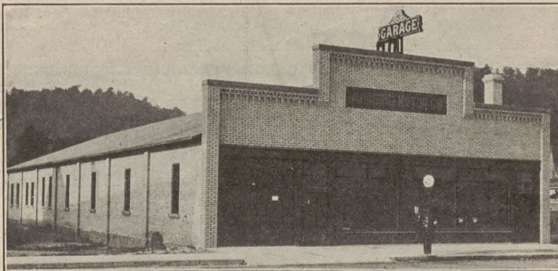
The Munising Motor Company's New Garage
